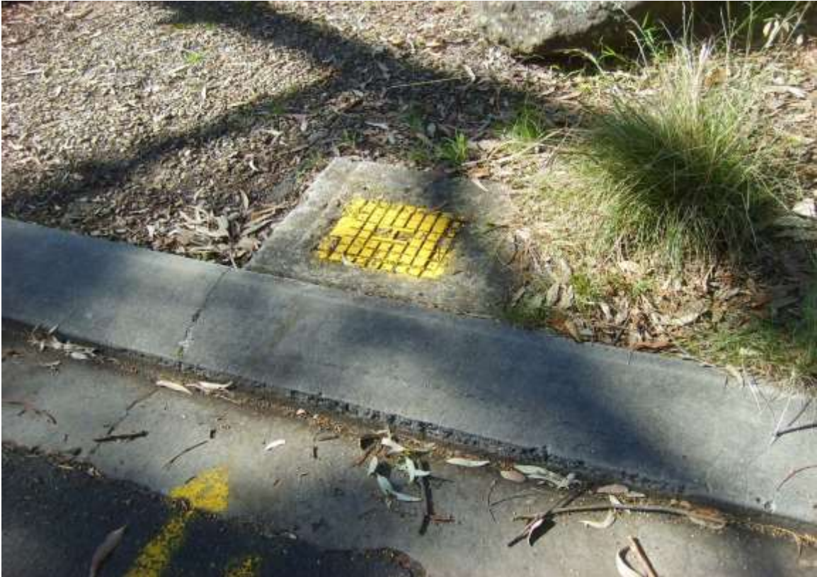
Photo 2 – Indicates the reticulated mains pressure fire hydrant located outside No. 123 Pacific Rd (Steve Brooks 2019)
