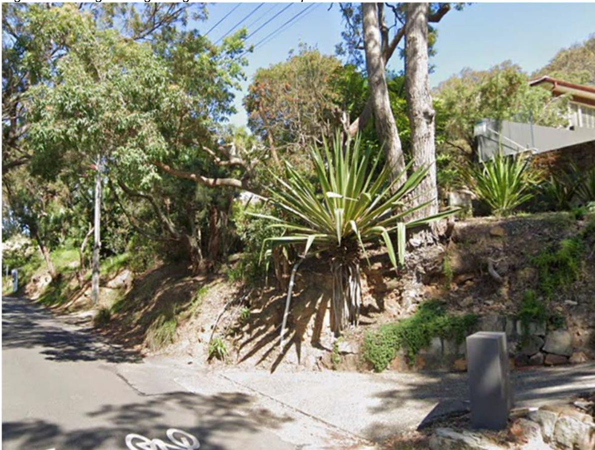
Image 4 - Showing existing failing stone wall and tree with exposed roots.
