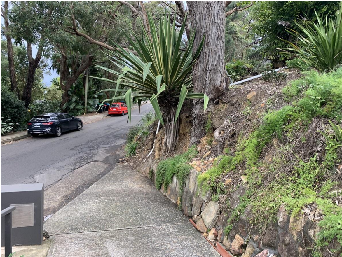
Image 3 - Showing existing failing stone wall to be replaced and tree to be removed.
