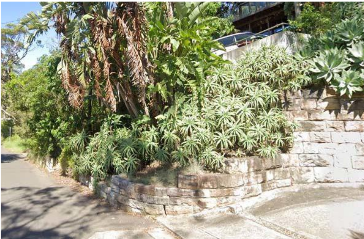
Image 2 - Existing stone retaining walls located on council verge and alongside driveways on Whale Beach Road.
