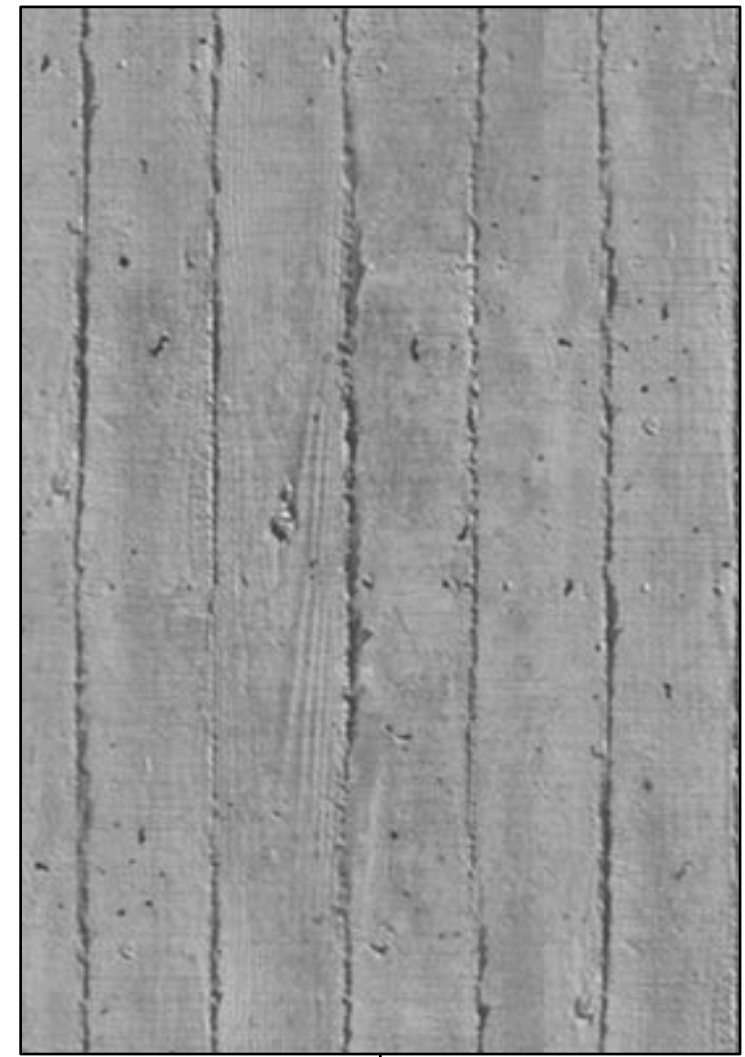
IN-SITU CONCRETE BOARD-MARKED VERTICAL 100MM
