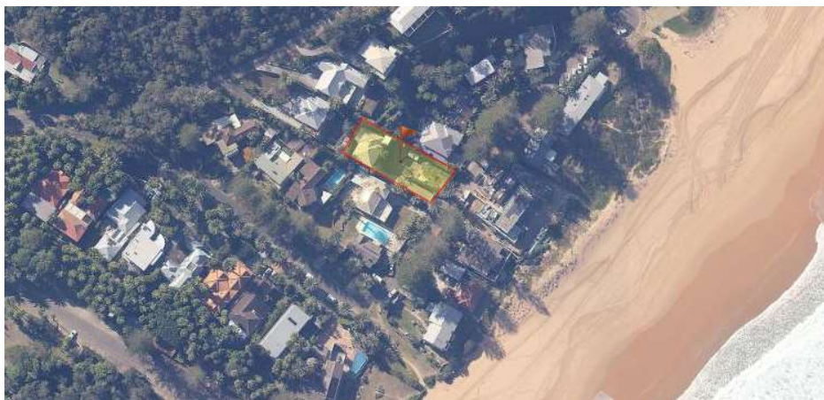
Photograph-1: Aerial photo of site and surrounds
