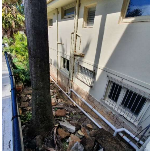
Photograph-5: Large tree located directly adjacent to the site boundary/concrete ramp. View looking south-east.
