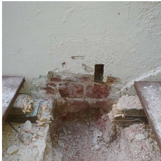
Photograph-12: TP1 excavation. View looking down west.
