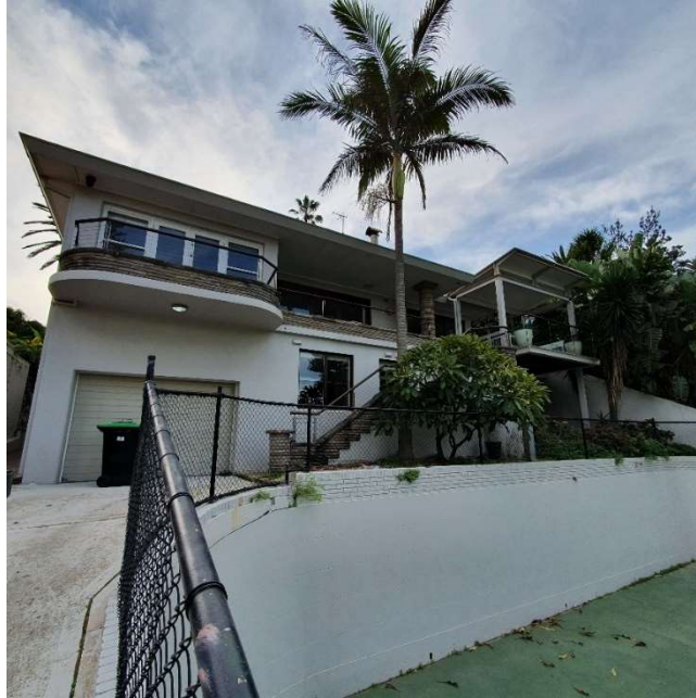
Photograph-3: Site-dwelling frontage. View looking north-west.
