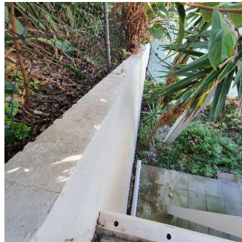
Photograph-7: Brick retaining wall along the north boundary. View looking down east.
