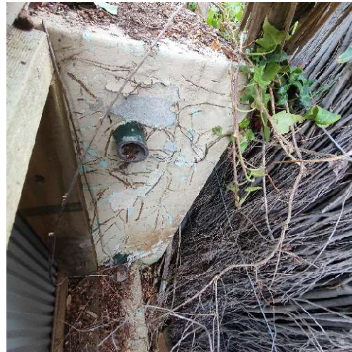
Photograph-9: Closer look to concrete pier. View looking south.
