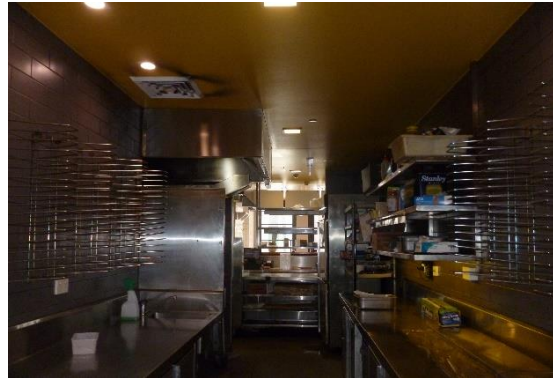
Figure 17: The kitchen area on the ground floor of The Ivanhoe Hotel
