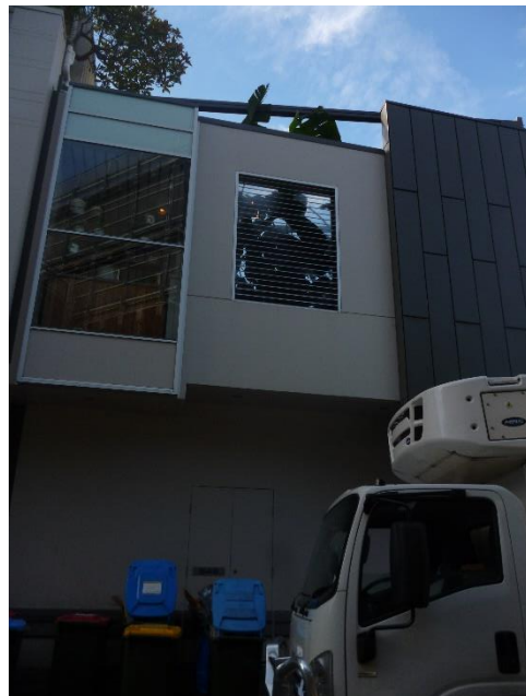
Figure 15: Rear (Market Place) elevation of 25 The Corso.
