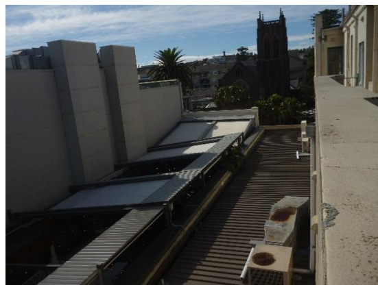
Figure 27: Rooftop view of 25 and 23 The Corso looking towards The Corso frontage
