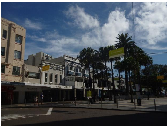
Figure 12: View of the subject site showing 19-21 (left), 23, 25 The Corso, and The Ivanhoe Hotel at the far end.
