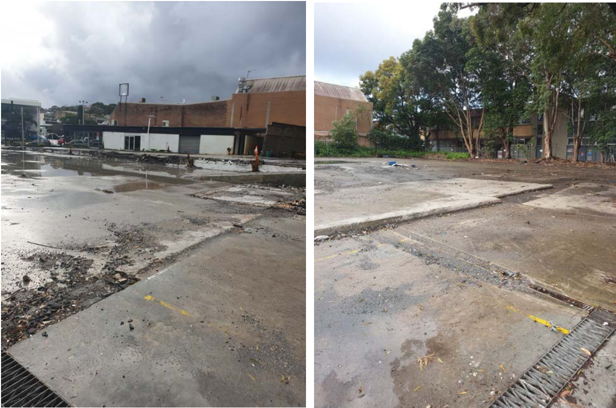
Figure 3 – Existing Warehouse at the Project Site
