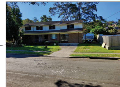
EXISTING DRIVEWAY AND EXISTING BUILDING, TO BE DEMOLISHED FOR PROPOSED DRIVEWAY AND HARDSTAND AREA
