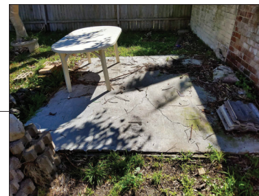
EXISTING CONDITION OF COUNCIL DRAINAGE ASSET TO BE RETAINED
