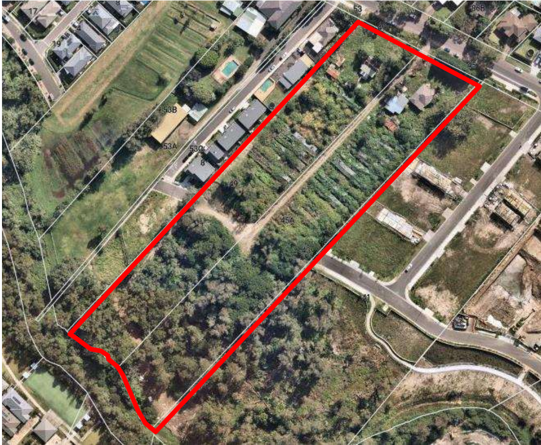
Figure 4: A closer aerial photo of the subject site. Note that Lorikeet Grove has not been constructed through the site, as indicated on mapping information within figure 2 .
