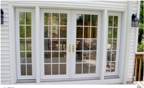
AFD ALUMINIUM FRENCH DOOR FRAME POWDERCOAT FINISH 'WHITE' OR SIMILAR WHERE MARKED ON ELEVATION.
