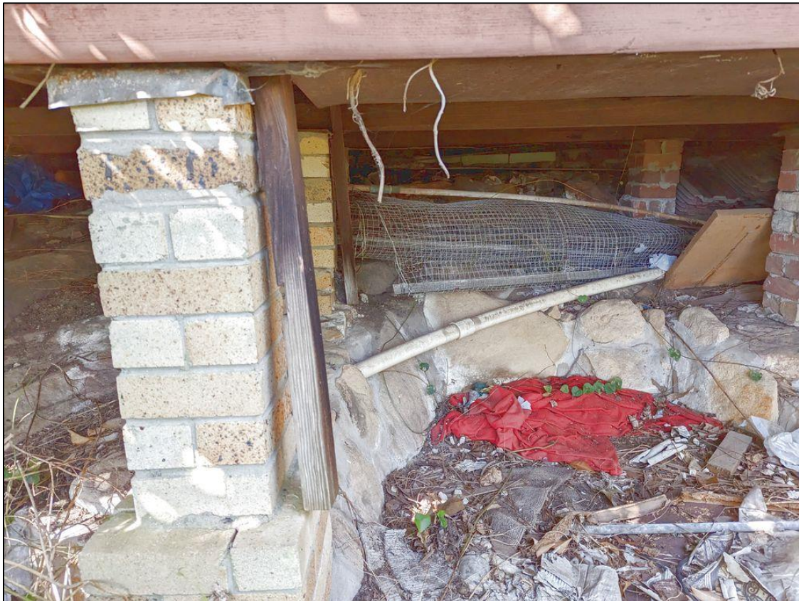
Photograph 14: Looking under the shed at 14 Gladys Avenue.
