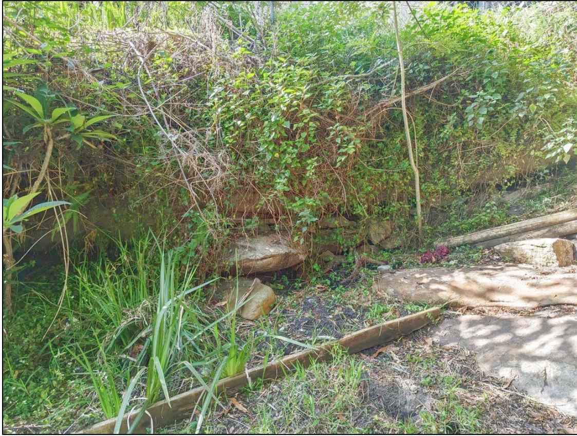
Photograph 5: Showing the area under the pool at 12 Gladys Avenue.
