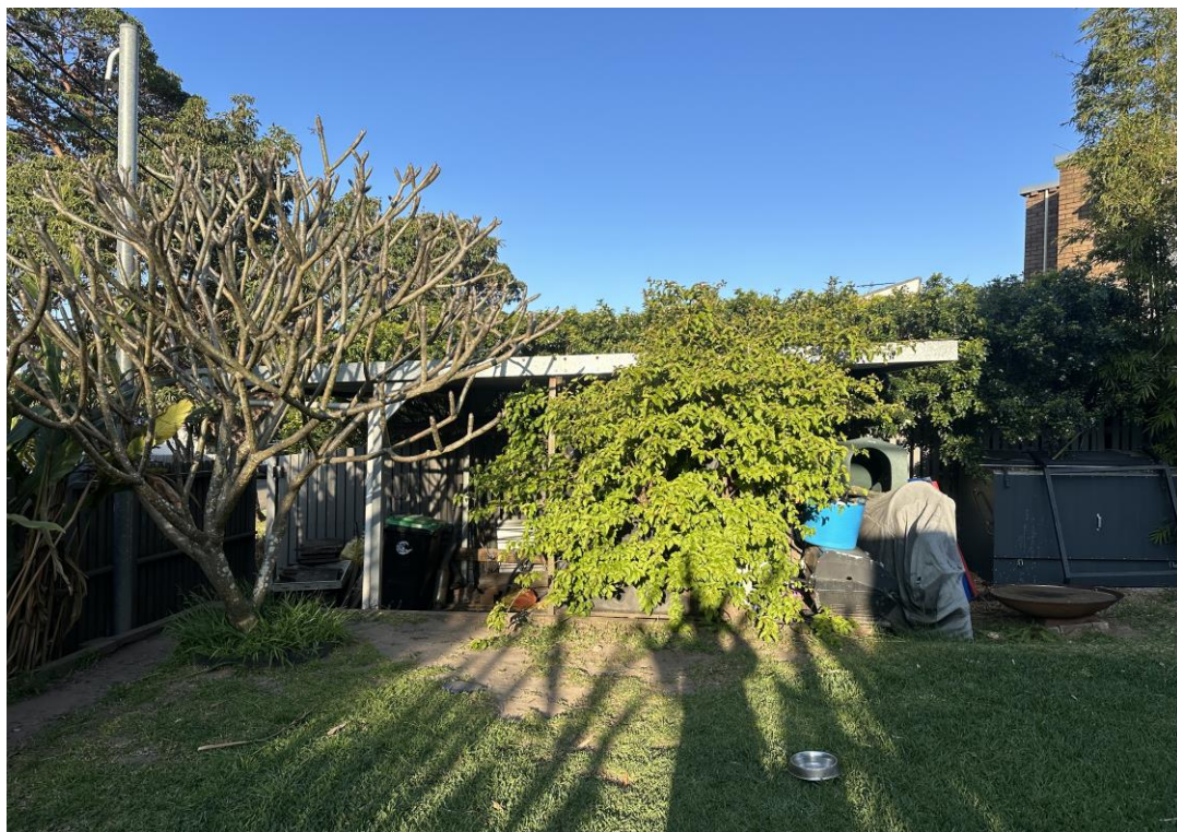
Figure 5. The existing carport, looking east.
