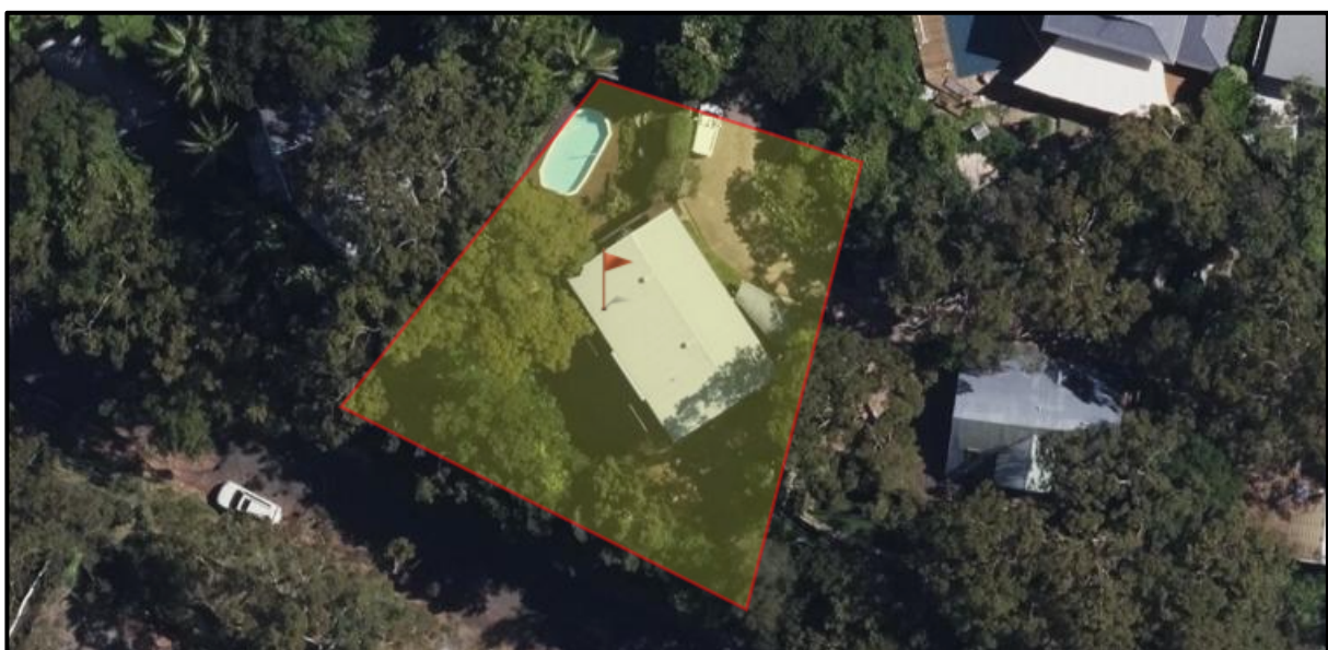
Figure 1. Site location – 12 Capua Place, Avalon Beach NSW (© SIX Maps NSW Gov)
