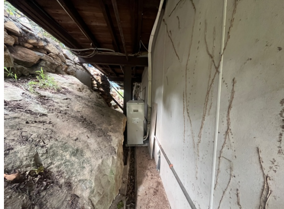
Photo 2: Sandstone outcropping on the northern side of the residence
