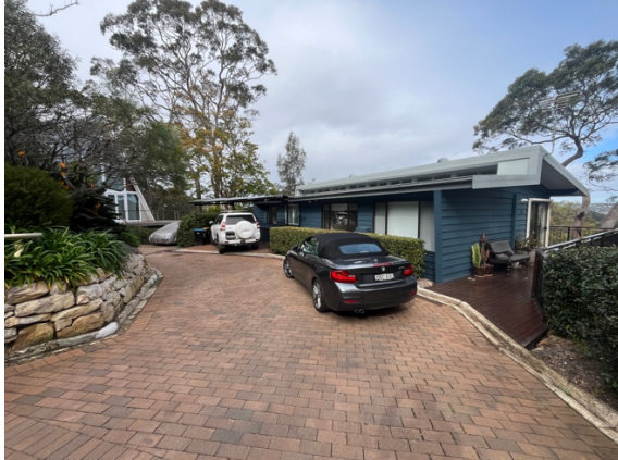
Photo 1: Right of carriageway access and residence frontage
