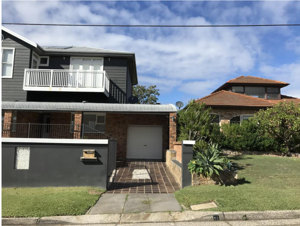
Fig 3: View of subject dwelling and its associated entry driveway and common western boundary with adjoining site at No 1 Summit Avenue, looking south from Summit Avenue
