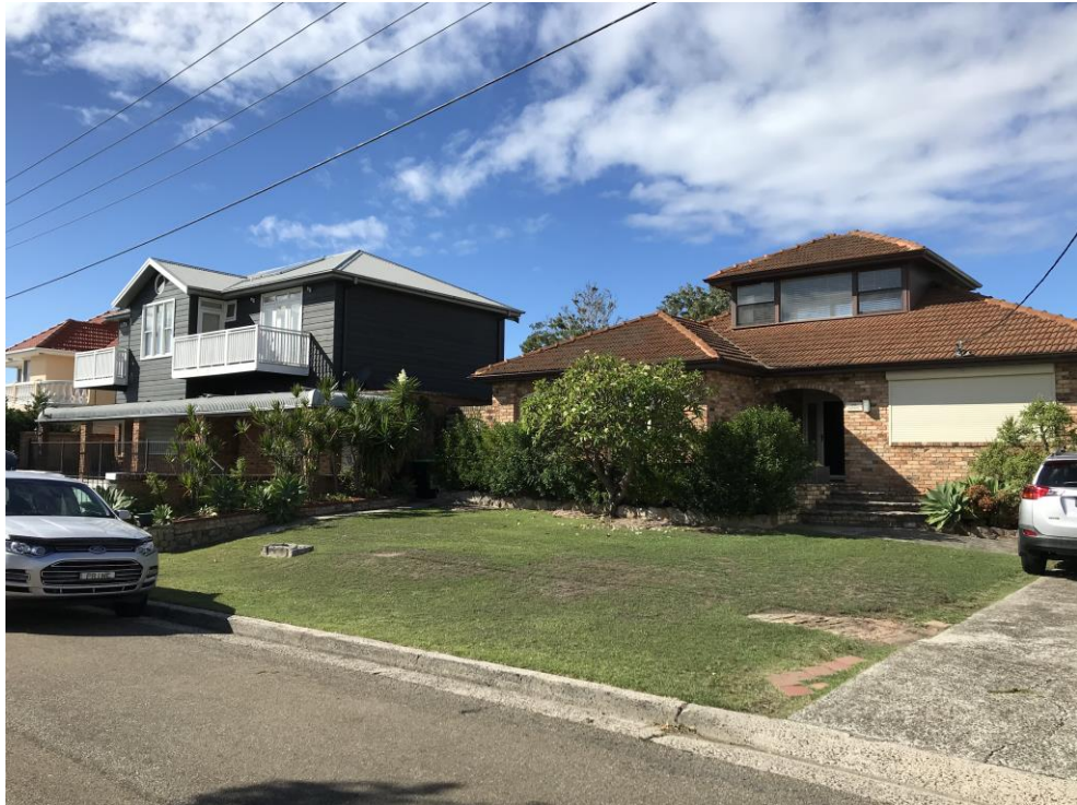
Fig 4: View of subject dwelling and the adjoining site at No 1 Summit Avenue, looking south-east from Summit Avenue
