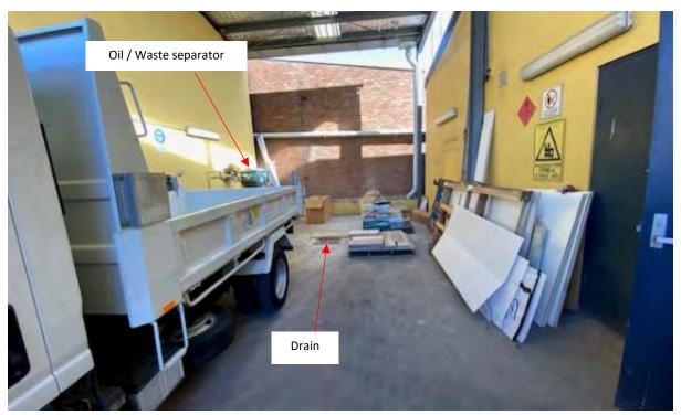
**Photograph 6:** Looking west towards the former vehicle car wash with locations of drain and oil / waste separator shown.
