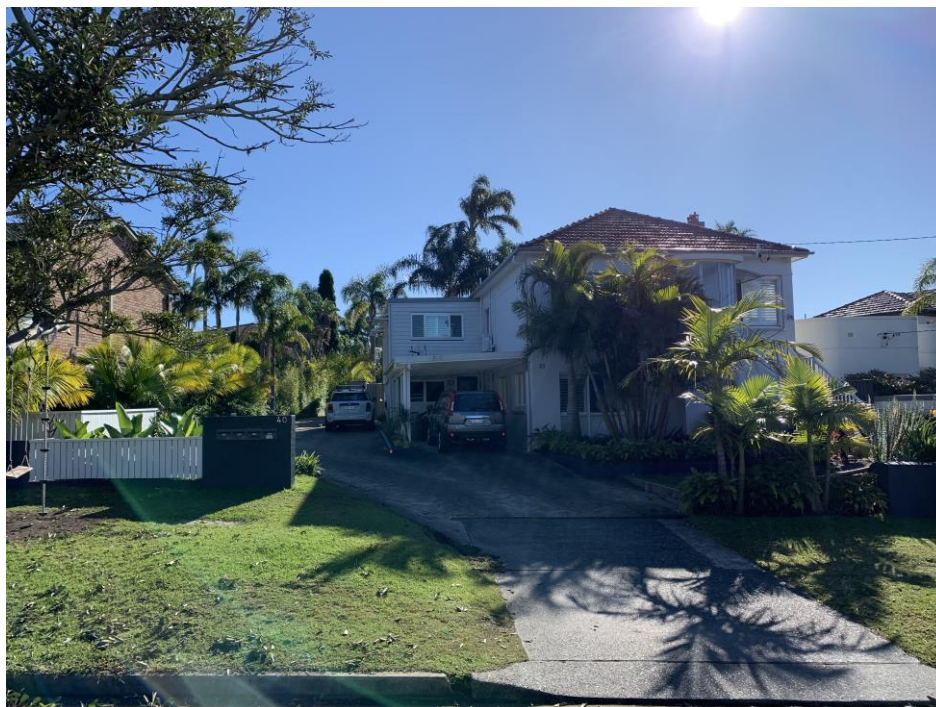
Fig 2: View of subject site as viewed from Serpentine Crescent, looking north
