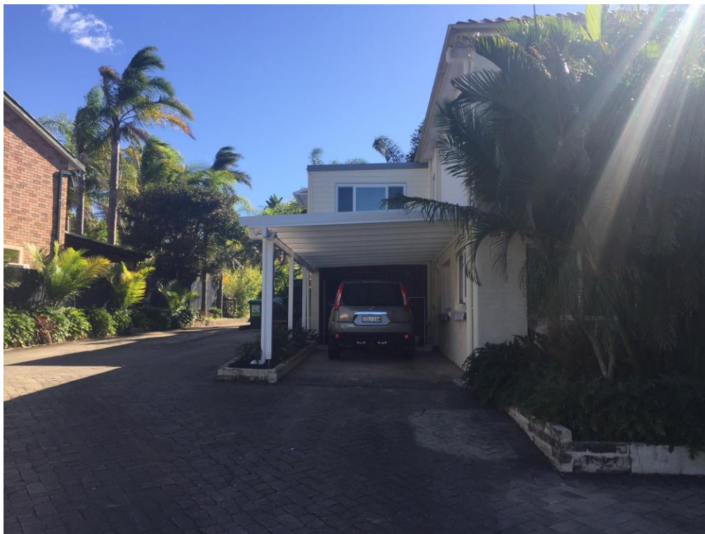
Fig 4: View of the existing ground floor level carport, with area at first floor level to be extended to provide and ensuite and walk in robe for the first floor level dwelling
