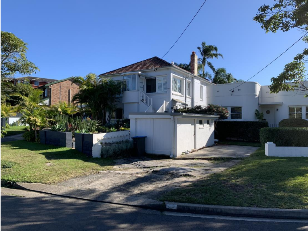
Fig 5: View of subject site and neighbouring dwelling at 42 Serpentine Crescent, looking north-west
