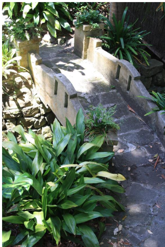
Photo 8 Stone bridge over drainage channel.
