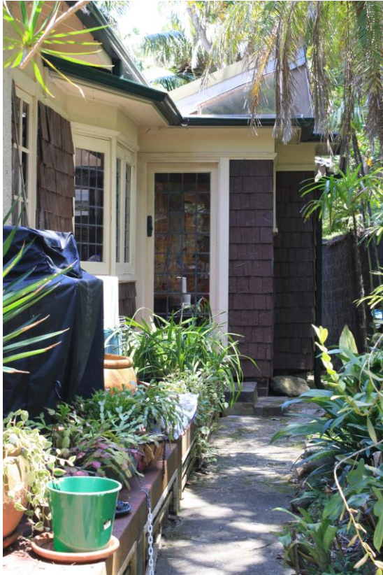
Photo 3 Rooflight over later rear addition.
