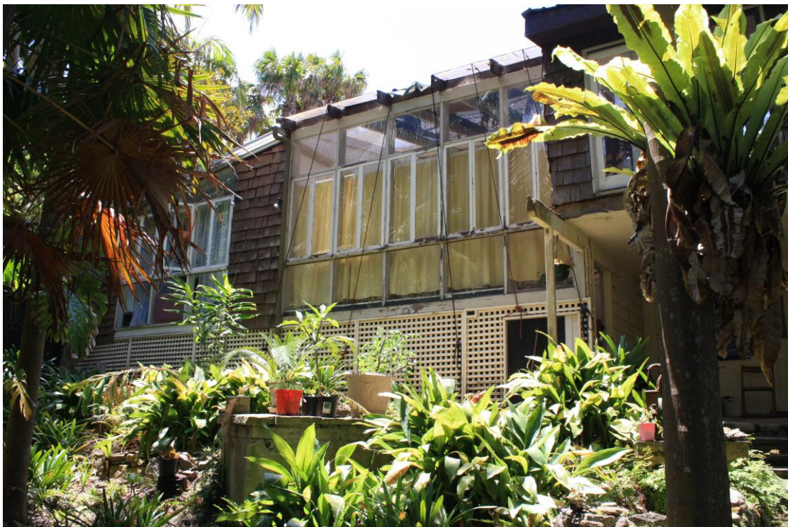
Photo 5 Rear addition to be demolished.
