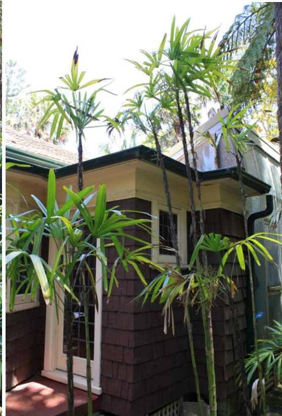
Photo 4 Present side entry to to be extended.
