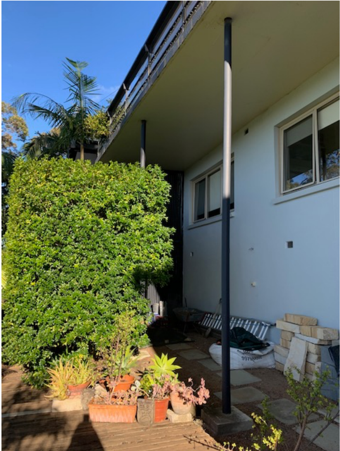
VIEW FROM EXISTING LEVEL 1 DECK TOWARDS SOUTH EAST BOUNDARY (shows existing structure of Level 3 balcony – concrete deck with supporting steel columns)
