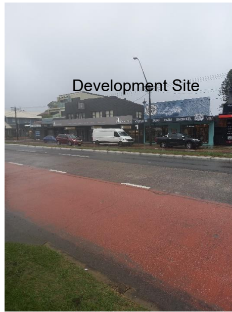
Pittwater Rd western lanes, note median strip directing uphill catchment overland flows to Ocean Grove (Barrenjoey Consulting Engineers pty ltd)
