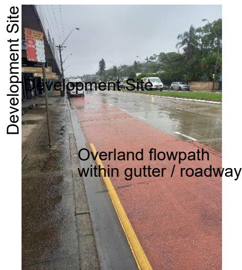
Pittwater Rd eastern lanes kerb / gutter (Barrenjoey Consulting Engineers Pty Ltd)
