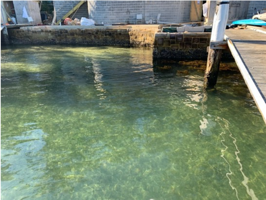
Figure 5 Sand beach plus rock rubble toe at the sandstone seawall.
