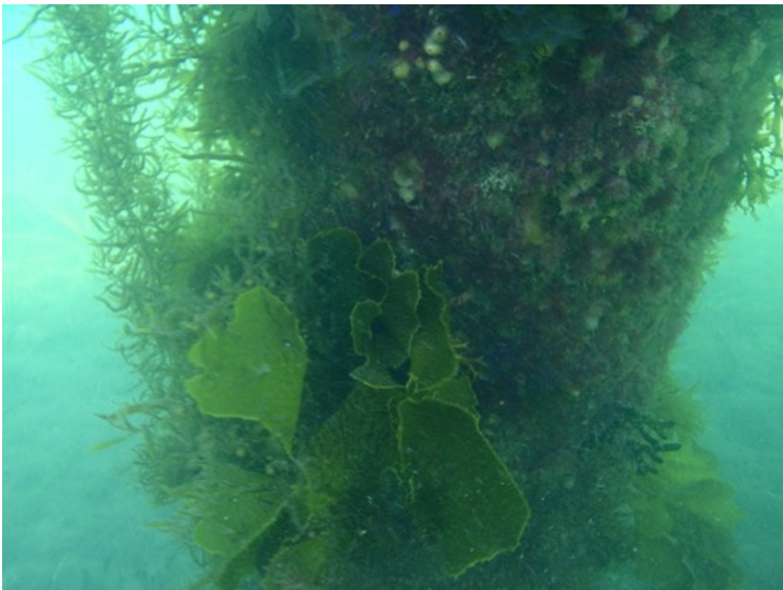
Figure 10 Kelp and Sargassum plus encrusting fauna attached to existing piles.
