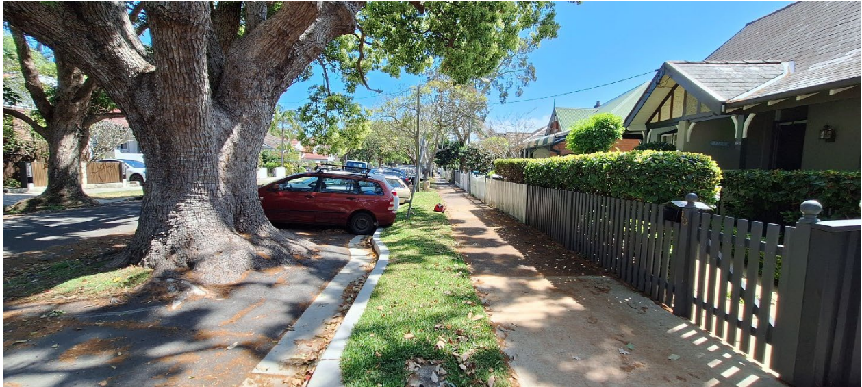
Photo 1: Recent gutter repair. T1 Camphor laurel within the road reserve. Proposed driveway beyond the tree. Photo looking west.
