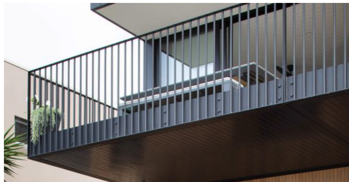
1 - STEEL BALUSTRADE POWDERCOAT FINISH 'BLACK' OR SIMILAR
