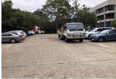
View of drilling at the car park
