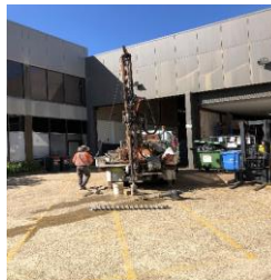
View of drilling at the front of warehouse
