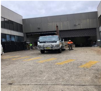
View of drilling at the front of warehouse
