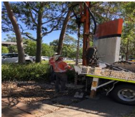
View of drill BH9/GW2
