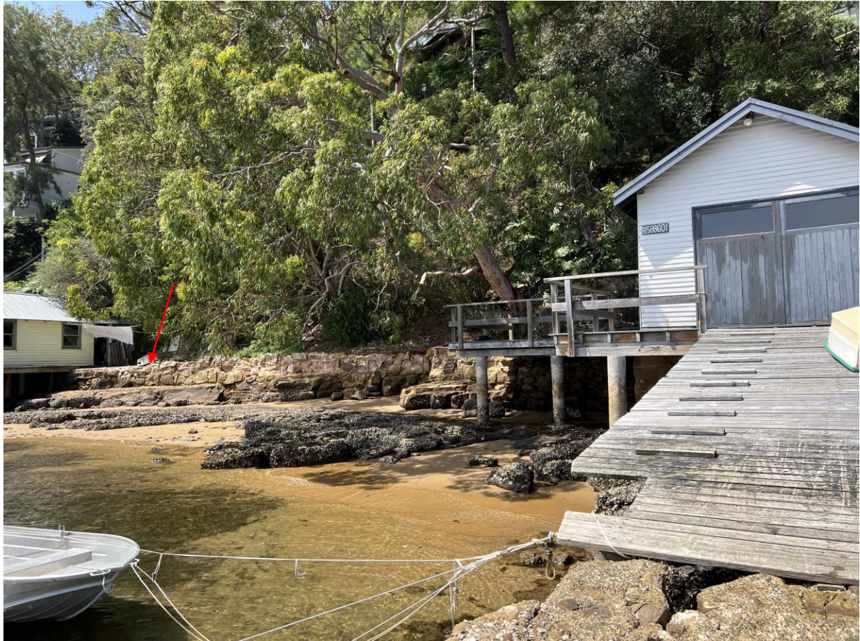
Figure 2: View of site (approximate northern extent at arrow) towards the ENE from foreshore on 7 March 2024 (southern boundary of site is to right of boatshed on right hand side of photograph)
