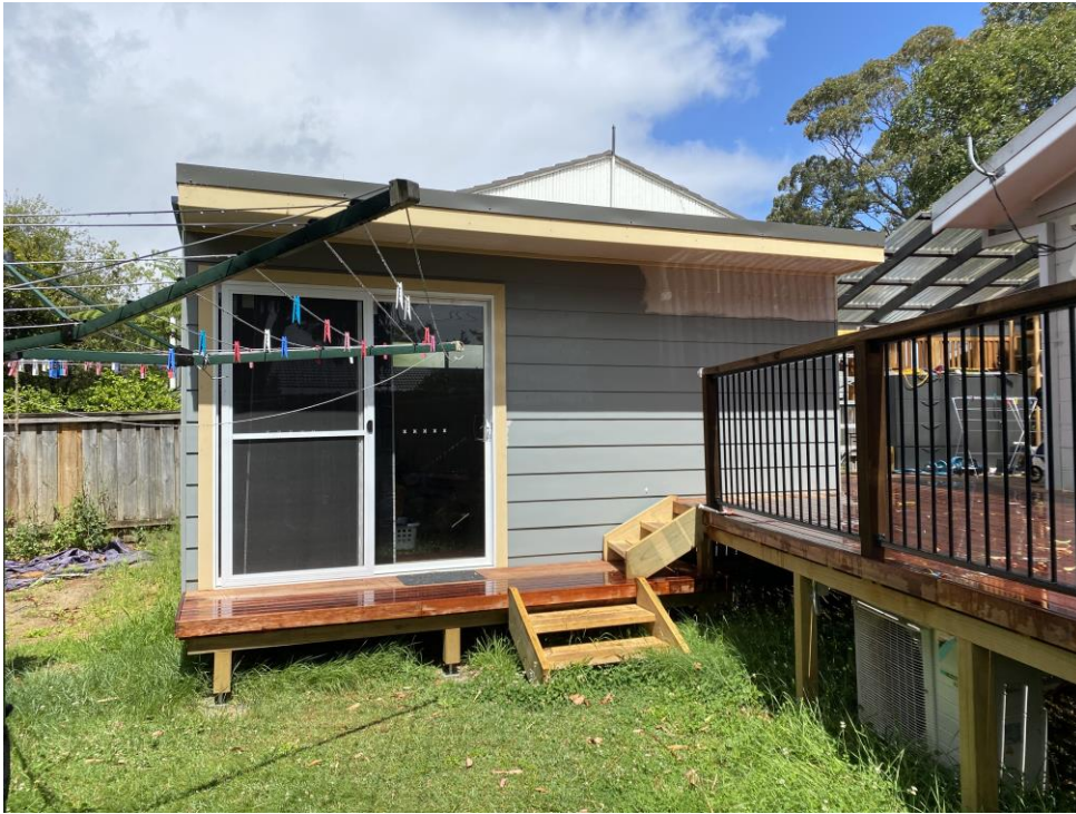
Figure 7. The existing shed built at the south eastern corner of the site
