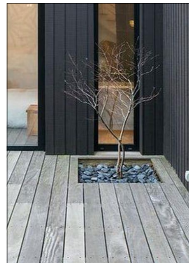
Selected dark wall cladding finish.
