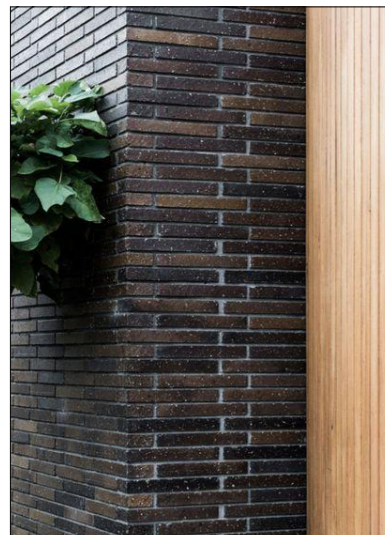
Selected, dark brick face brickwork.
