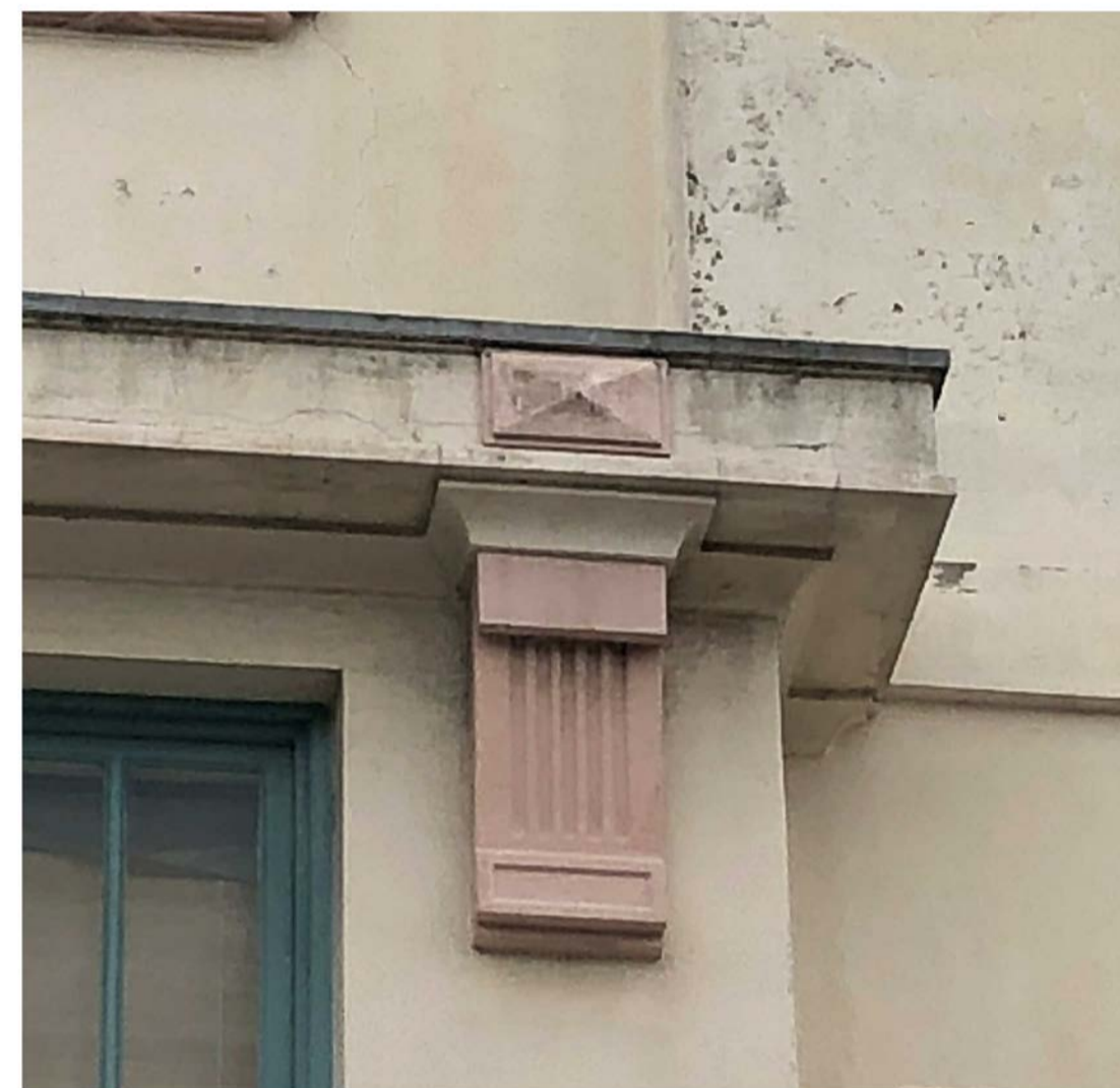
Open up and investigate cracking to pediment. Rectify cracking to structural engineer and heritage architect's advice and reinstate rendered detail to match original.
