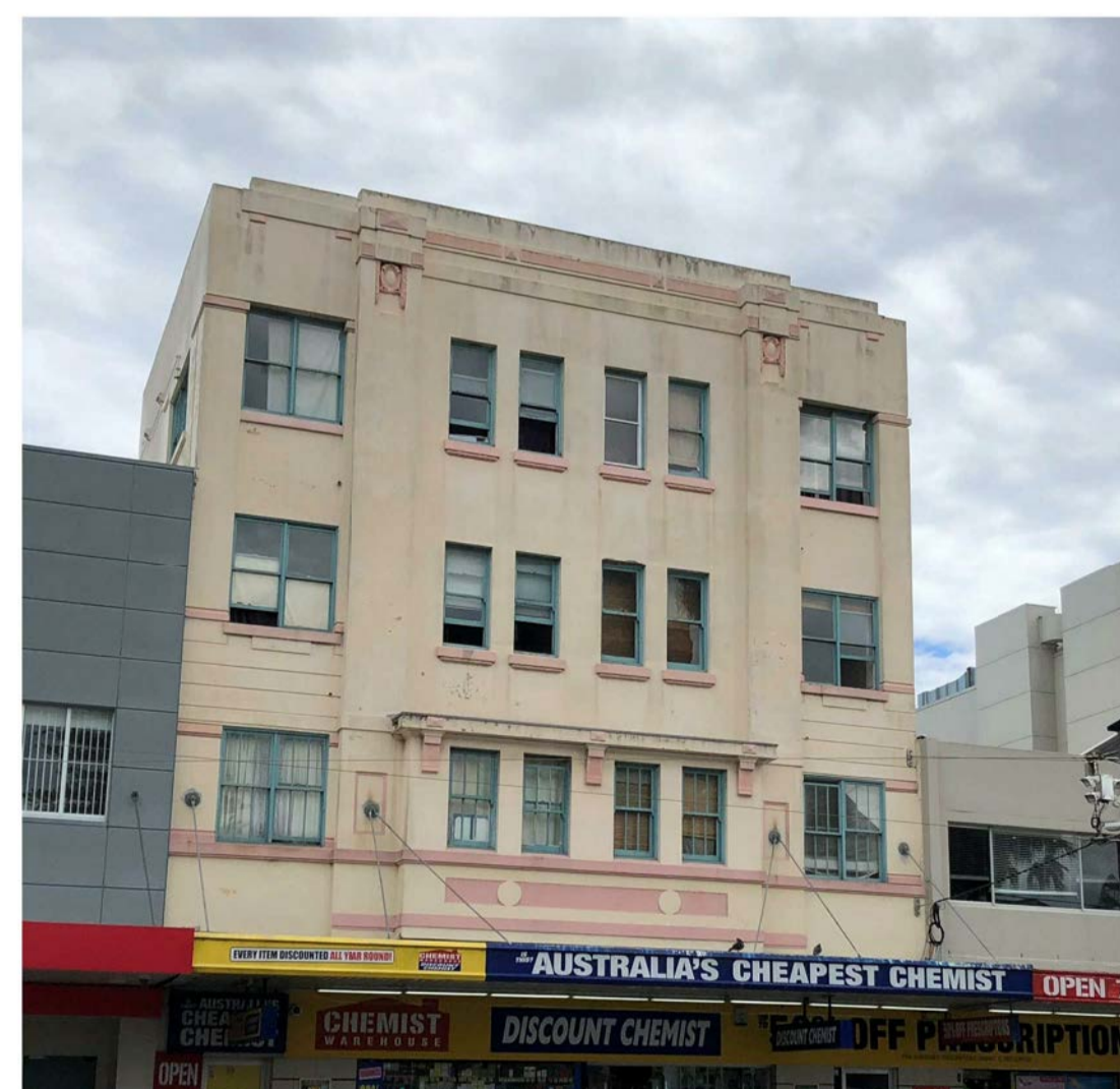
Allow to repaint entire façade and masonry returns to The Corso in heritage colour scheme based on paint scrape evidence performed on site once access to façade is provided. Paint shall be Dulux Acratex Acraseal or similar to heritage architect's approval.
