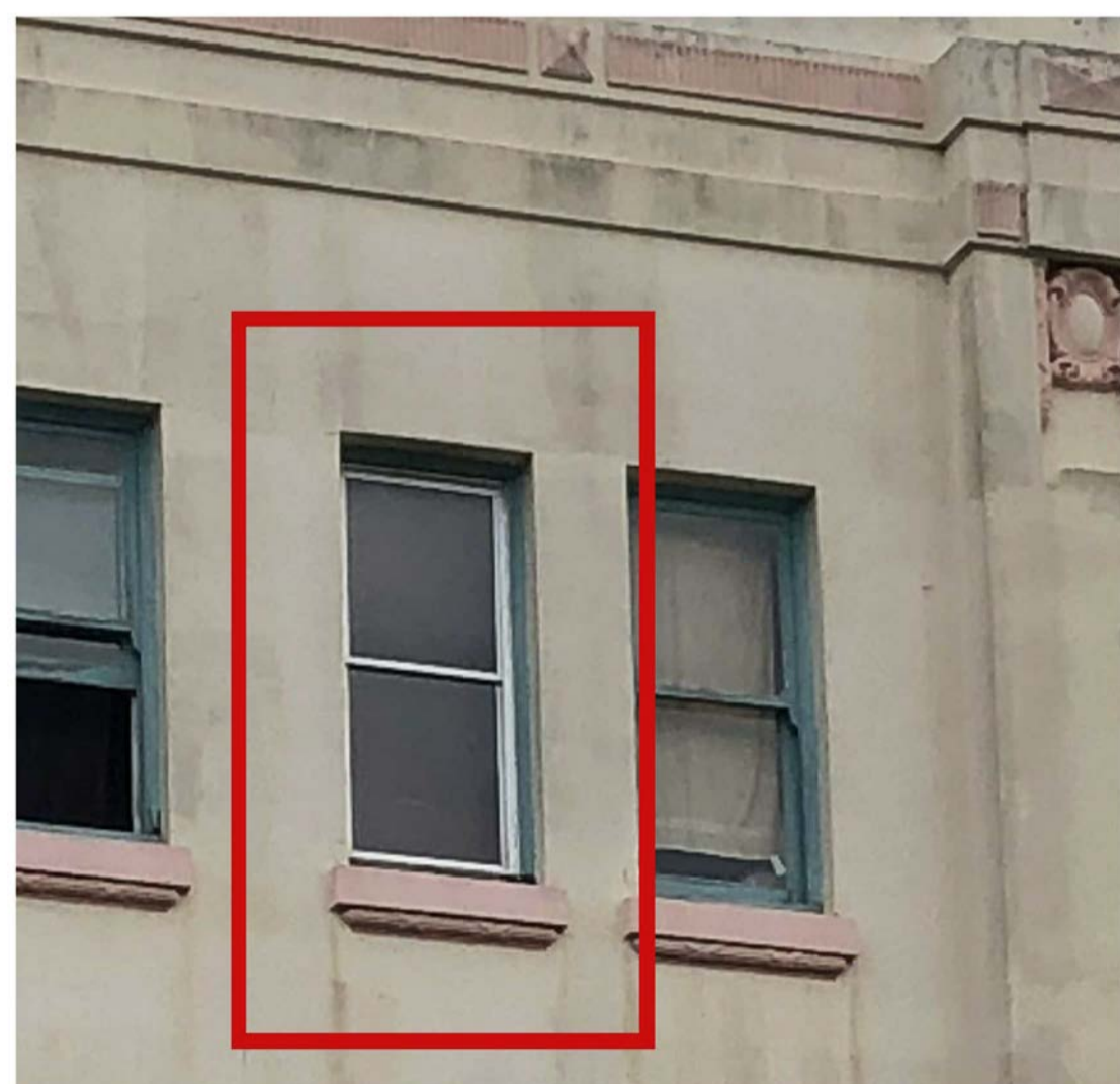
Reconstruct window to match original detailing.
