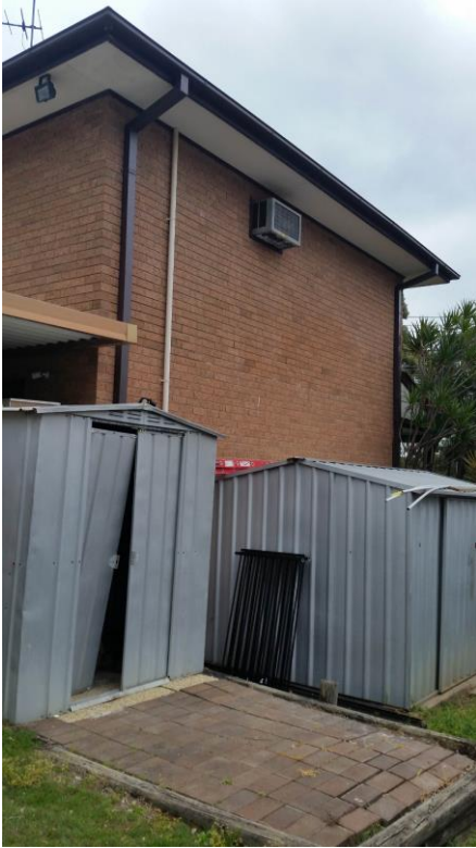
Looking along eastern setback area. Location of proposed addition
