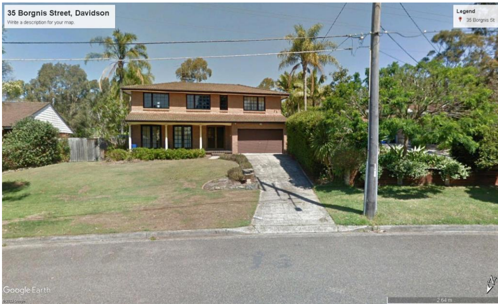
Looking at No.35 from Borgnis Street
