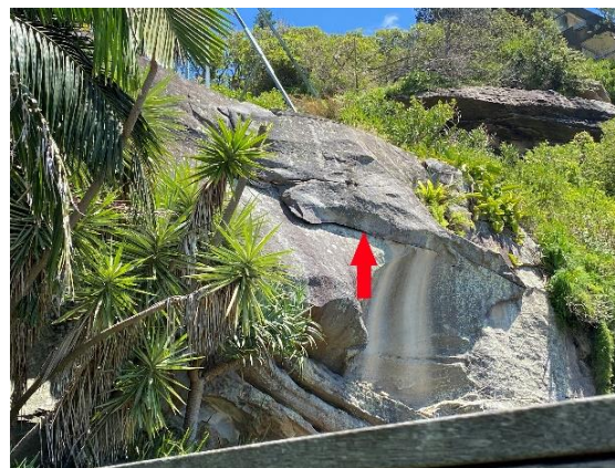
Spalling and fractured rock near cliff crest.
