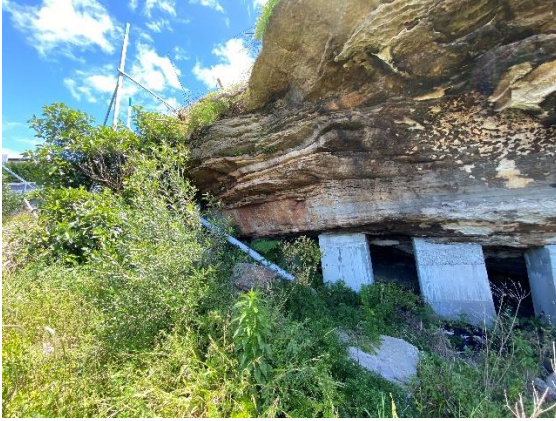
Outcrop cliff and underpinning at north-wets corner of No. 2
