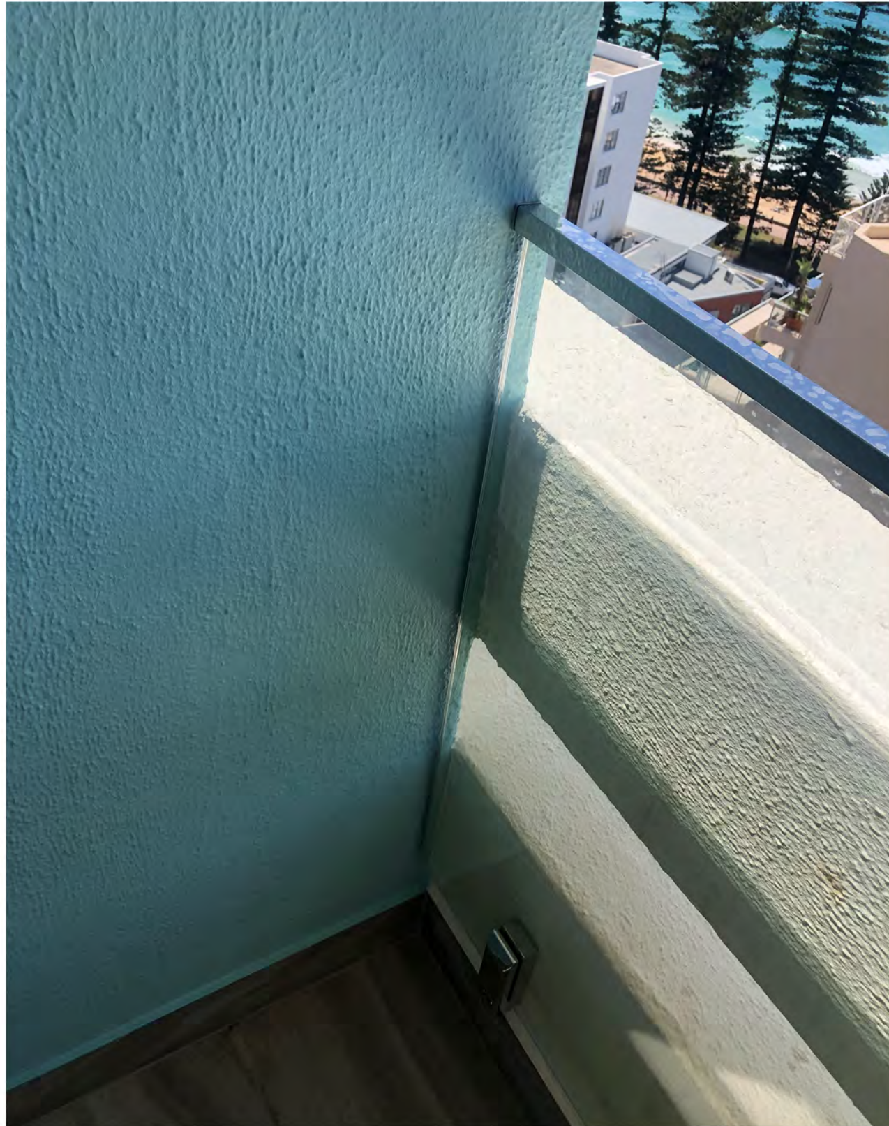
PHOTOS OF SAMPLE FIXING TO LOWER HOB AND GLASS BALUSTRADE
