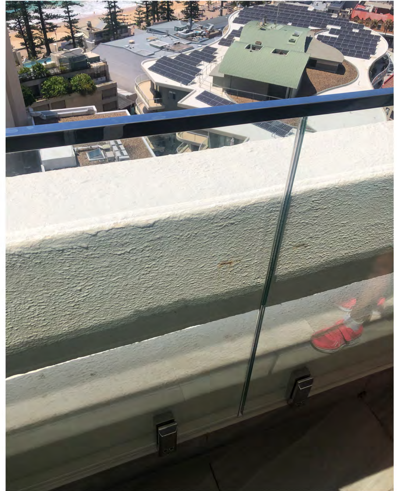
PHOTOS OF SAMPLE FIXING TO LOWER HOB AND GLASS BALUSTRADE
