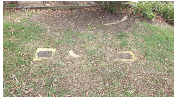
Reticulated water supply in pathway
