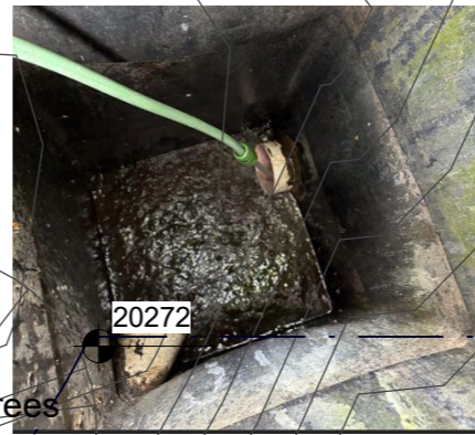
Photo: testing Storm water pit with hose
