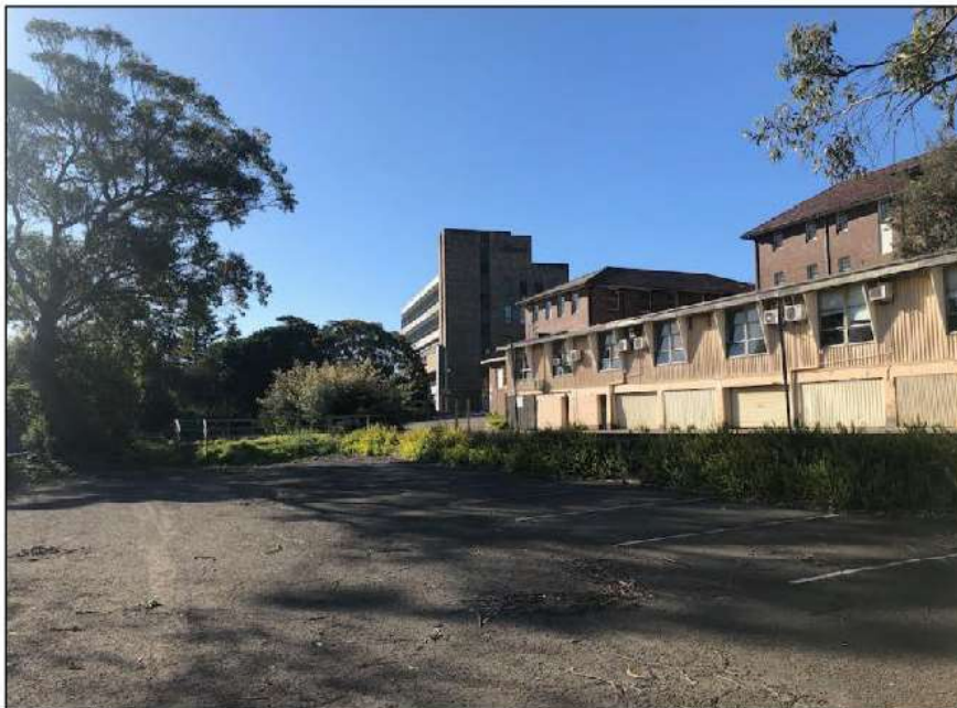
Figure 4 – View of the South Wing and Open Car Park Source: Mecone
