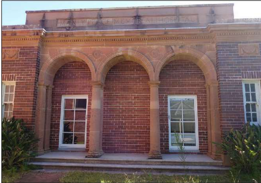
Figure 5 – Historic Building facade Located Within the Site Source: Mecone
