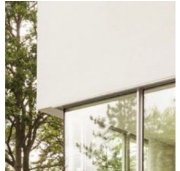
WD-01 - ALUMINIUM WINDOWS RB-01 - RENDERED CONCRETE BLOCK
