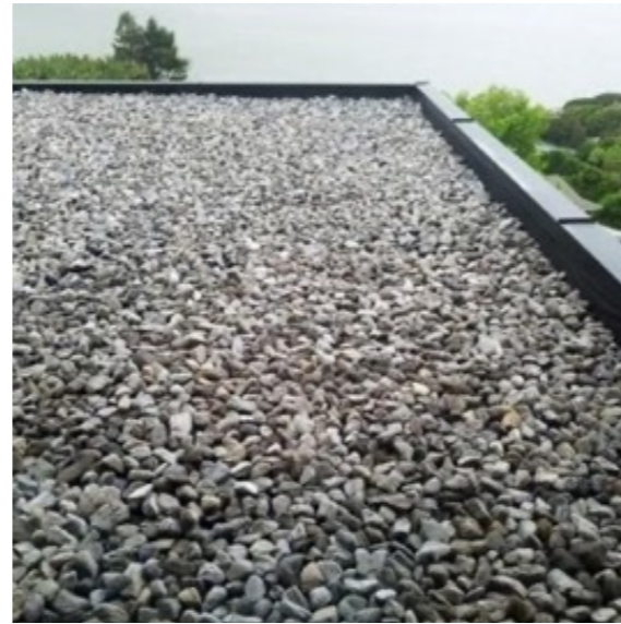
RF-01 - MEMBRANE / BALLASTED ROOF
