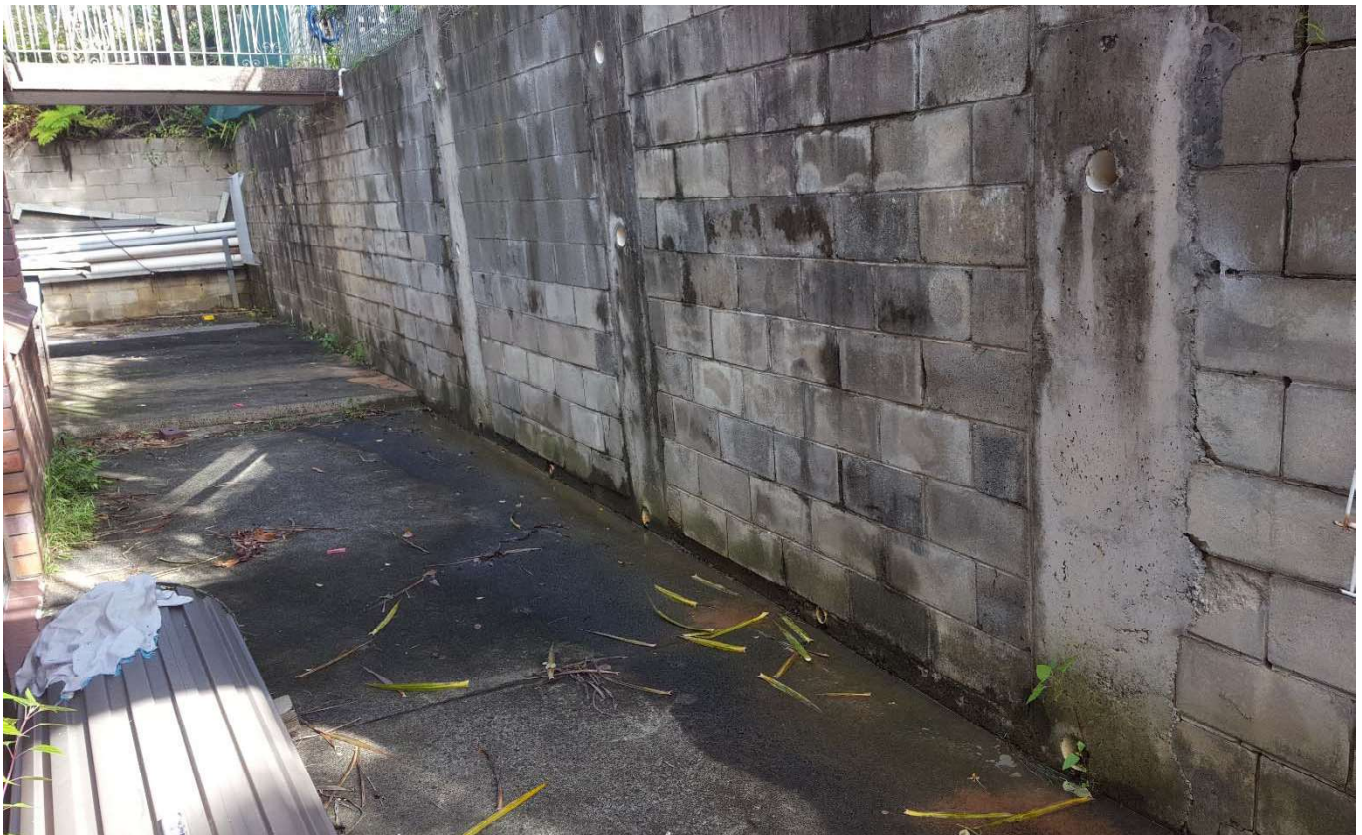
Figure 5 – Retaining wall and water ponding / seepage behind the existing house. Note: Seepage through wall joints. The high volume of seepage suggests that the excavation is close to the geological interface between Hawkesbury Sandstone and Newport Formation.
