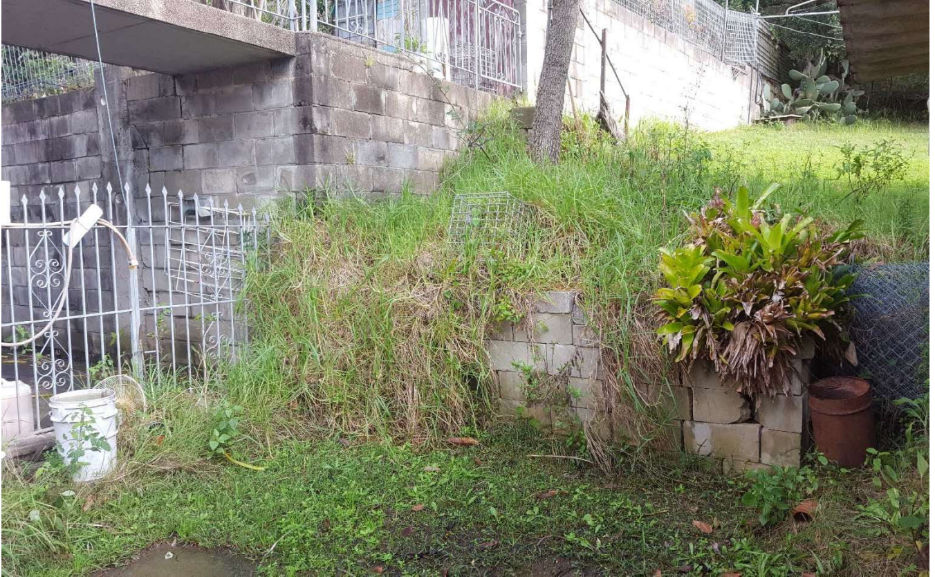
Figure 4 – Retaining walls, structures and slope behind existing house –central portion of land. Note: Ponding of water on the ground, seepage through the wall joints, movement of wall blocks.
