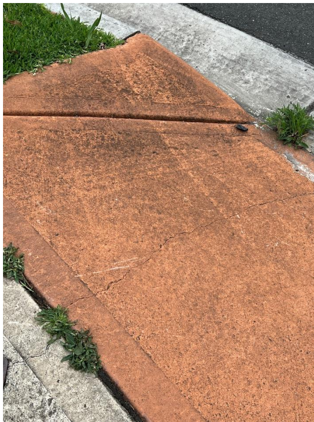
Figure 80 – Crack is evident to the layback.
