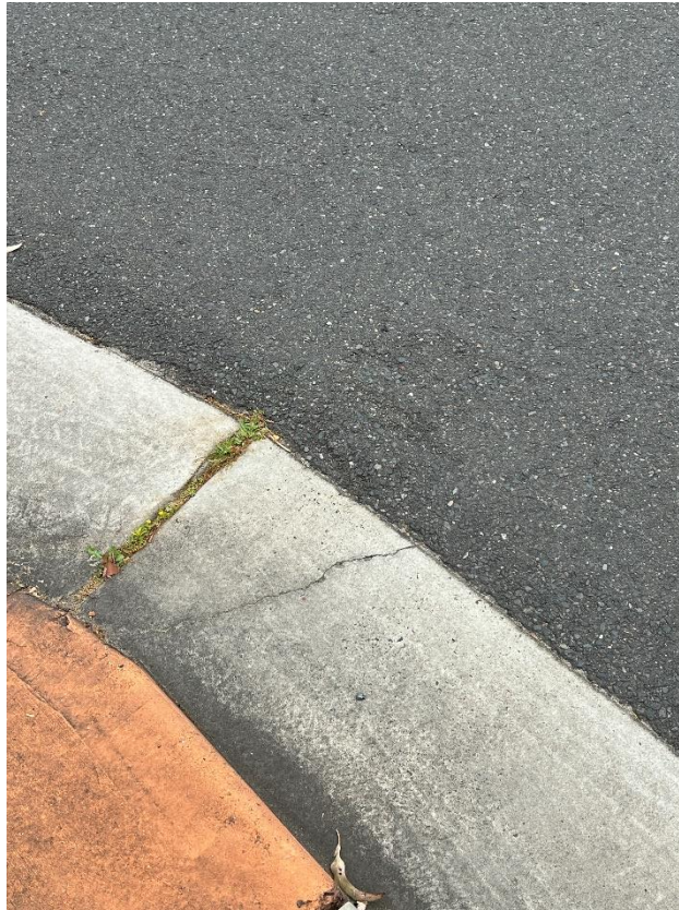
Figure 75 – Crack is evident to the layback.
