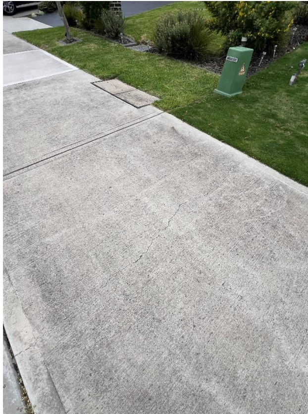
Figure 31 – Crack is evident to the footpath.
