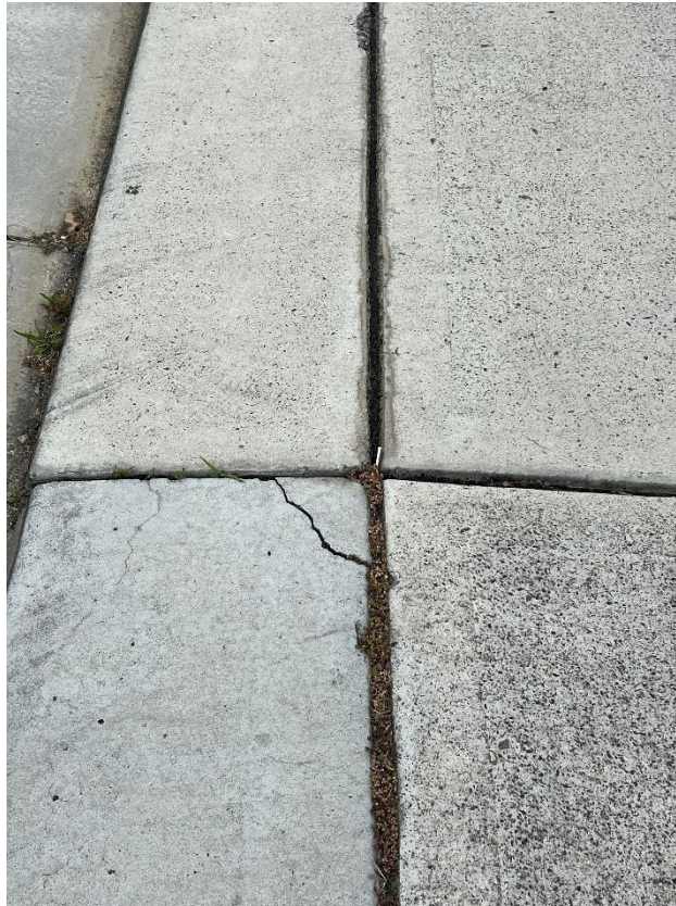
Figure 121 – Crack is evident to the layback.
