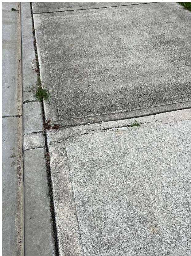
Figure 18 – Crack is evident to the footpath.
