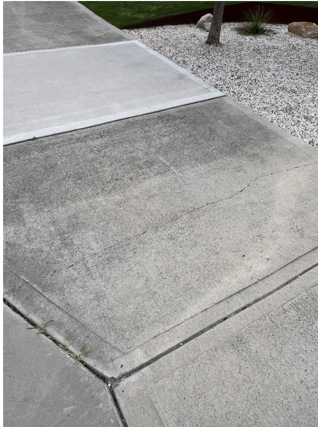
Figure 25 – Crack is evident to the footpath.
