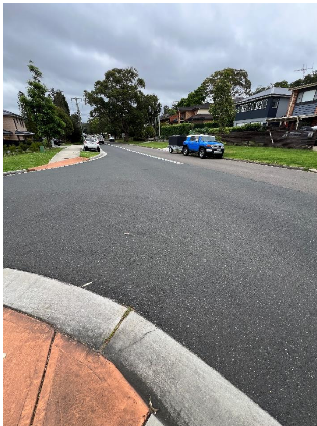
Figure 74 - Crack is evident to the layback.
