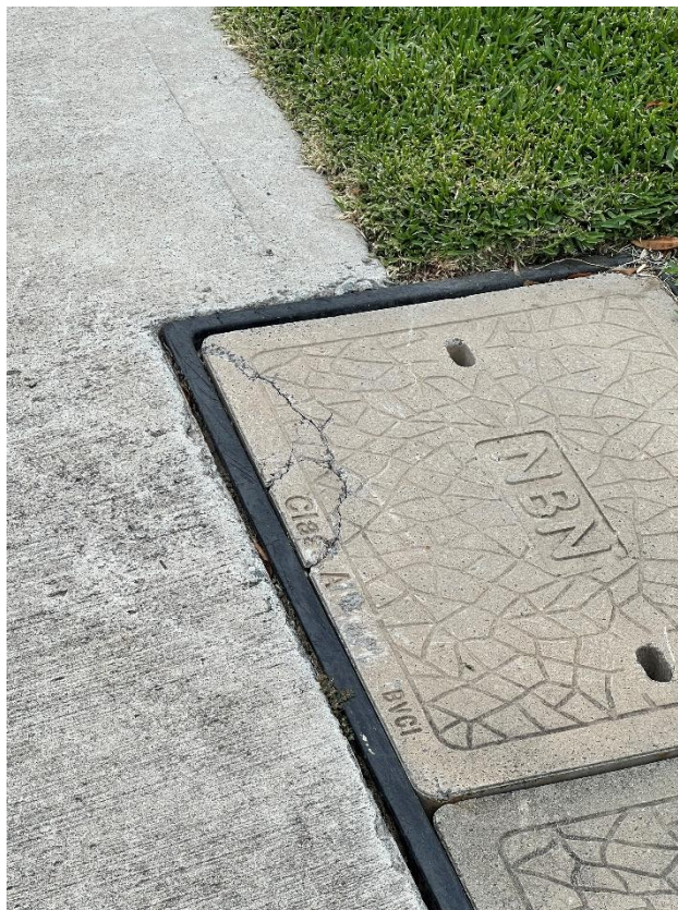
Figure 30 – Crack is evident to the pit.
