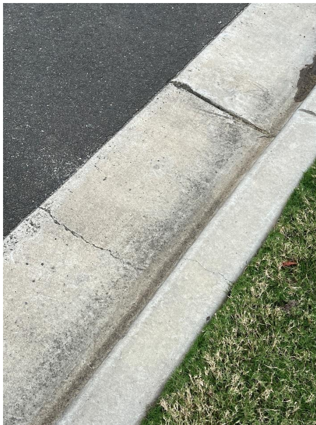
Figure 114 – Crack is evident to the kerb.
