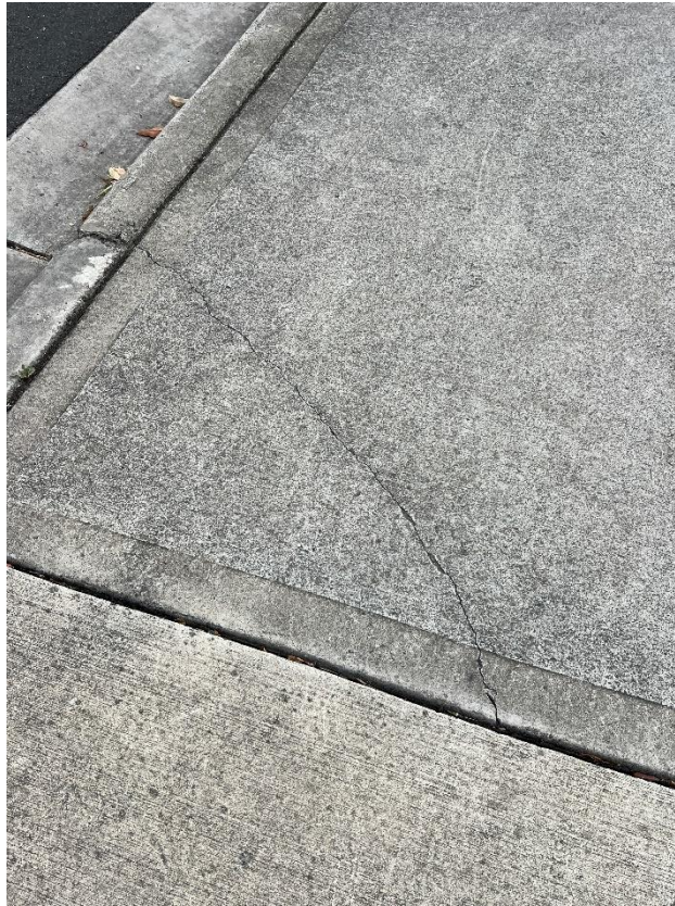
Figure 65 – Crack is evident to the footpath.
