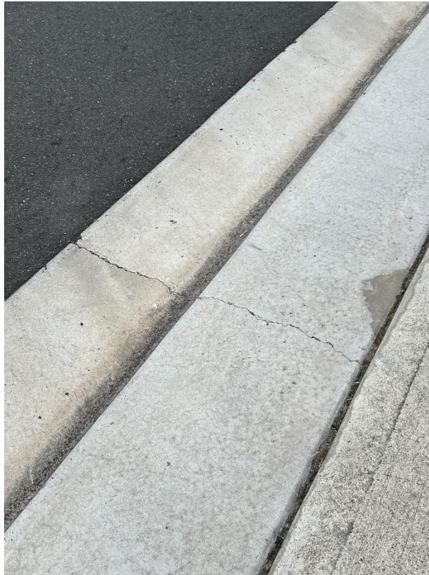
Figure 53 – Crack is evident to the layback.
