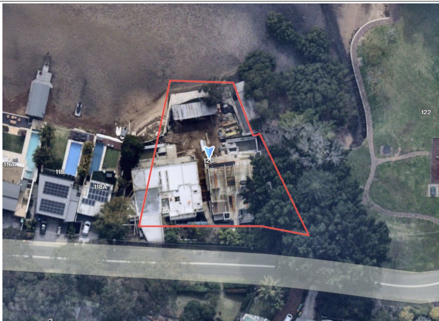
Figure 4 Aerial Image with the site delineated in red. Source: Near Map 4 August 2024
