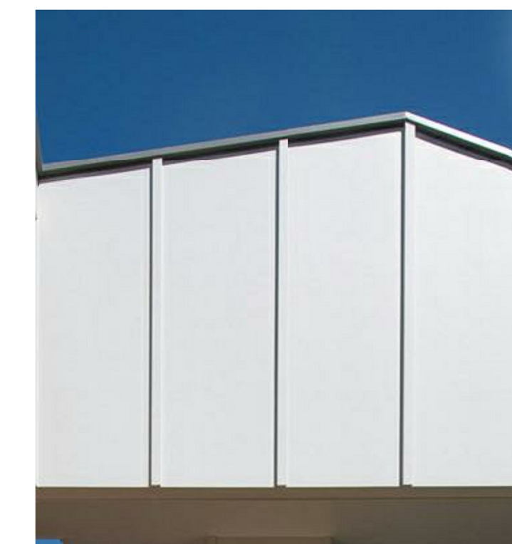
VERTICAL EXPRESSED CLADDING PANEL
