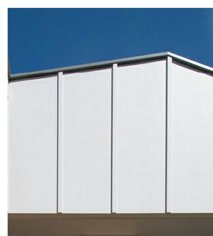
VERTICAL EXPRESSED CLADDING PANEL
