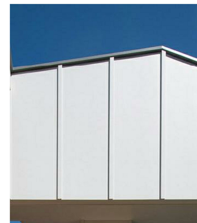
VERTICAL EXPRESSED CLADDING PANEL
