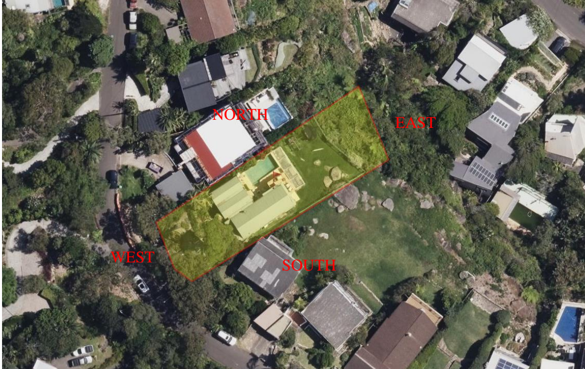
Photograph 1: Aerial photo of site and surrounds
