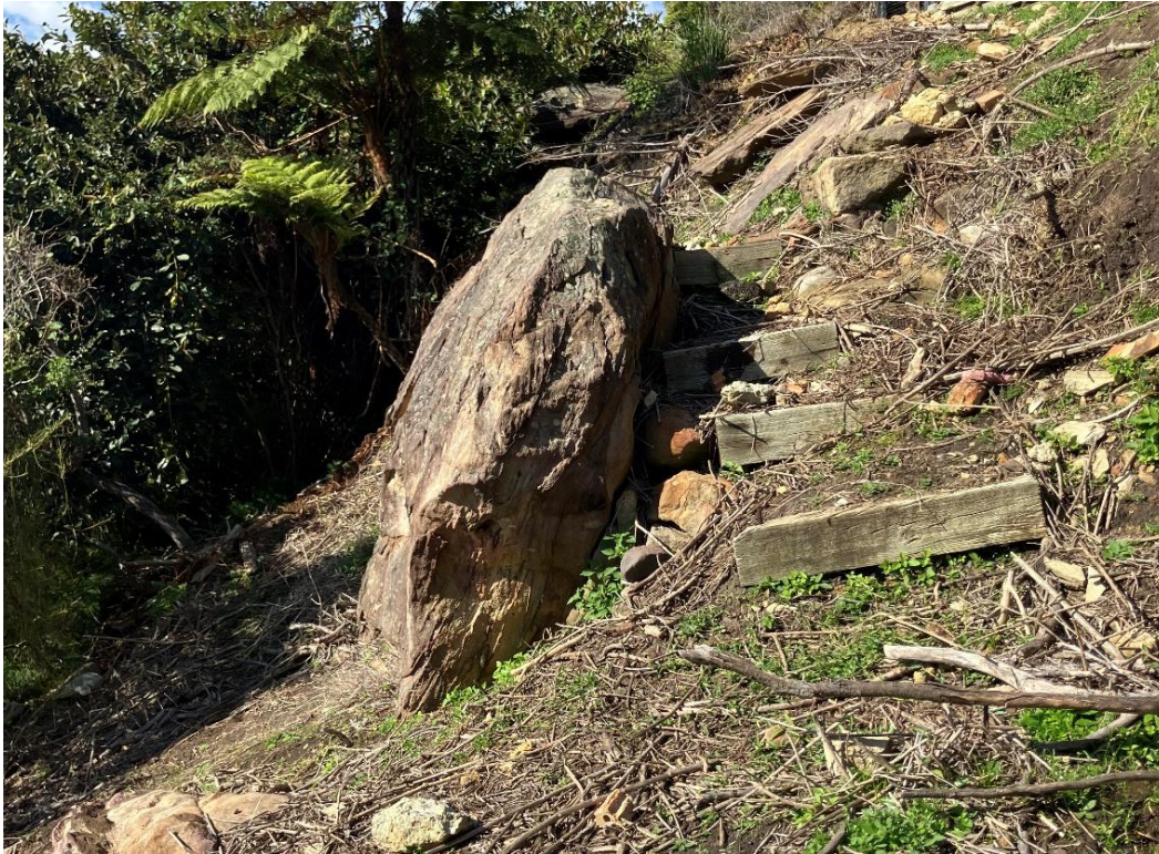
Photograph 4: View of the detached sandstone boulder within the rear garden, looking broadly south
