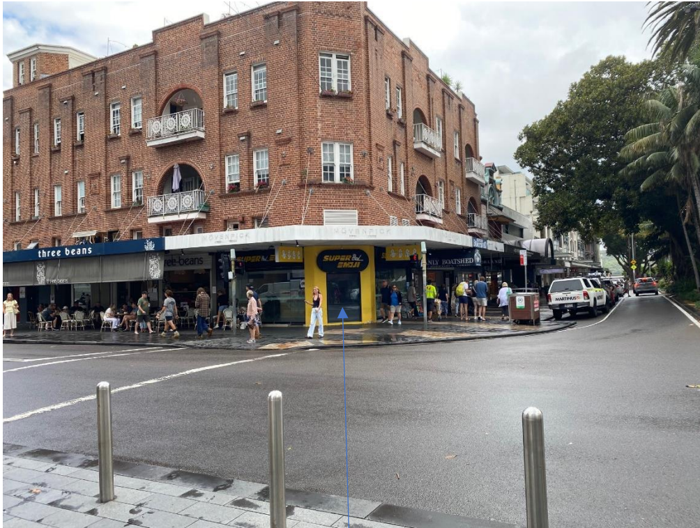
Photograph of 38-42 The Corso, Manly – Lot 8 the subject tenancy is located on the ground floor corner
