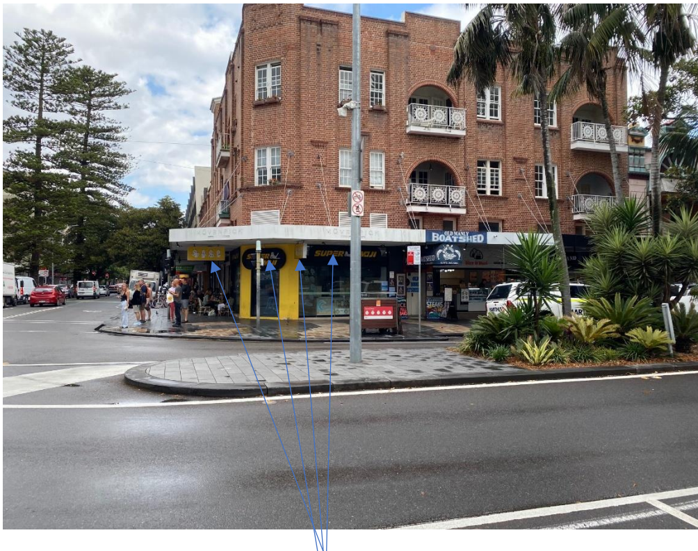
Photograph of the site – note existing signs to be replaced with new business logos
