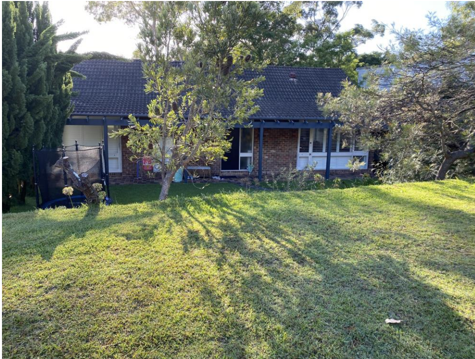
Figure 8. The front of the property, looking east
