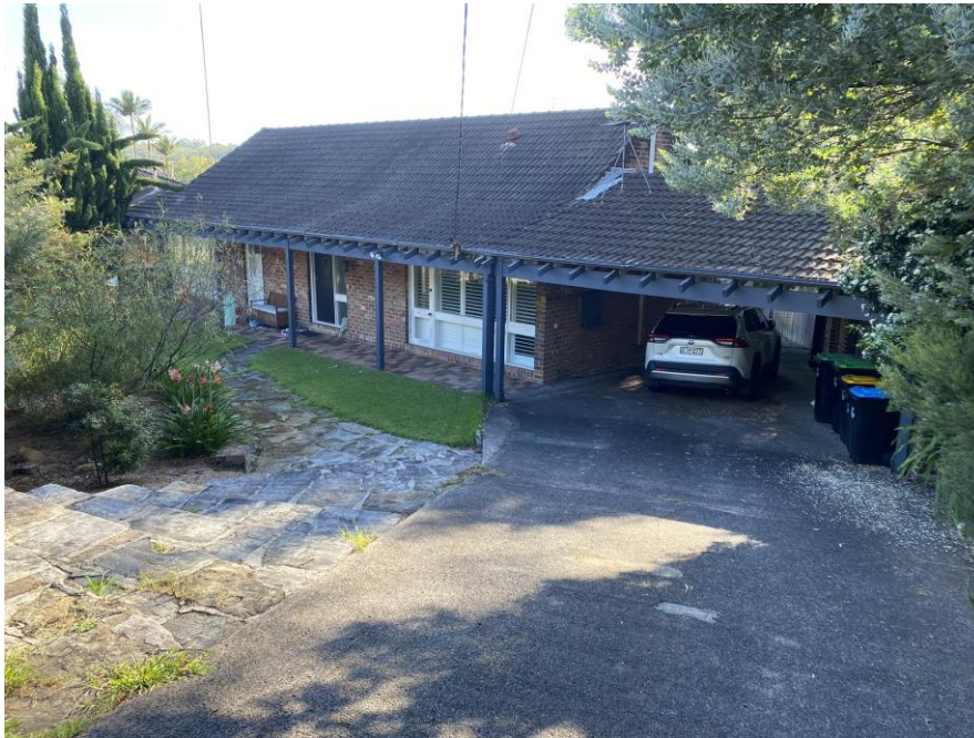
Figure 4. The western (front) elevation of the existing dwelling, looking north-east from Tipperary Avenue
