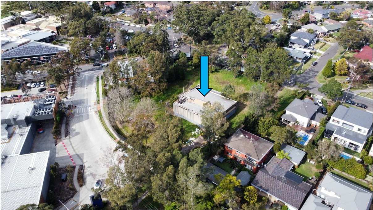
Figure 3: The site looking to the south-west (Prior to demolition)
