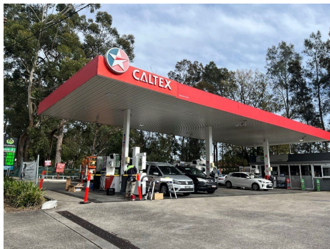
Figure 12: Petrol station adjoining the site to the east
