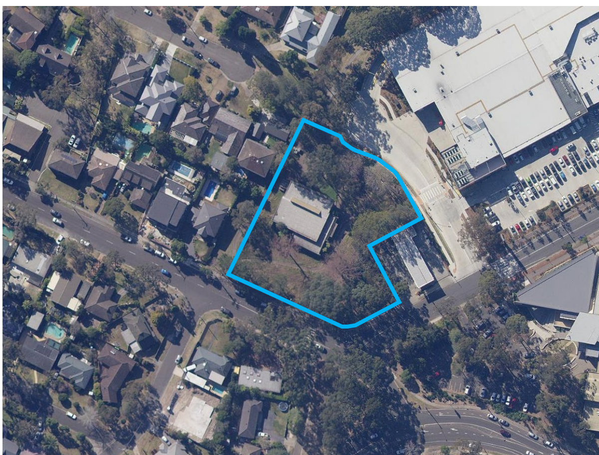
Figure 1: The site and surrounding area (Prior to demolition)
