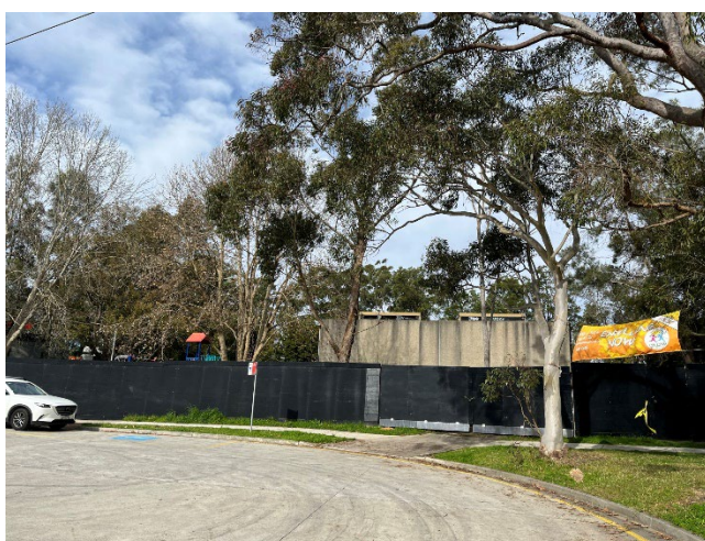
Figure 9: The site from Glenrose Place (Prior to demolition)
