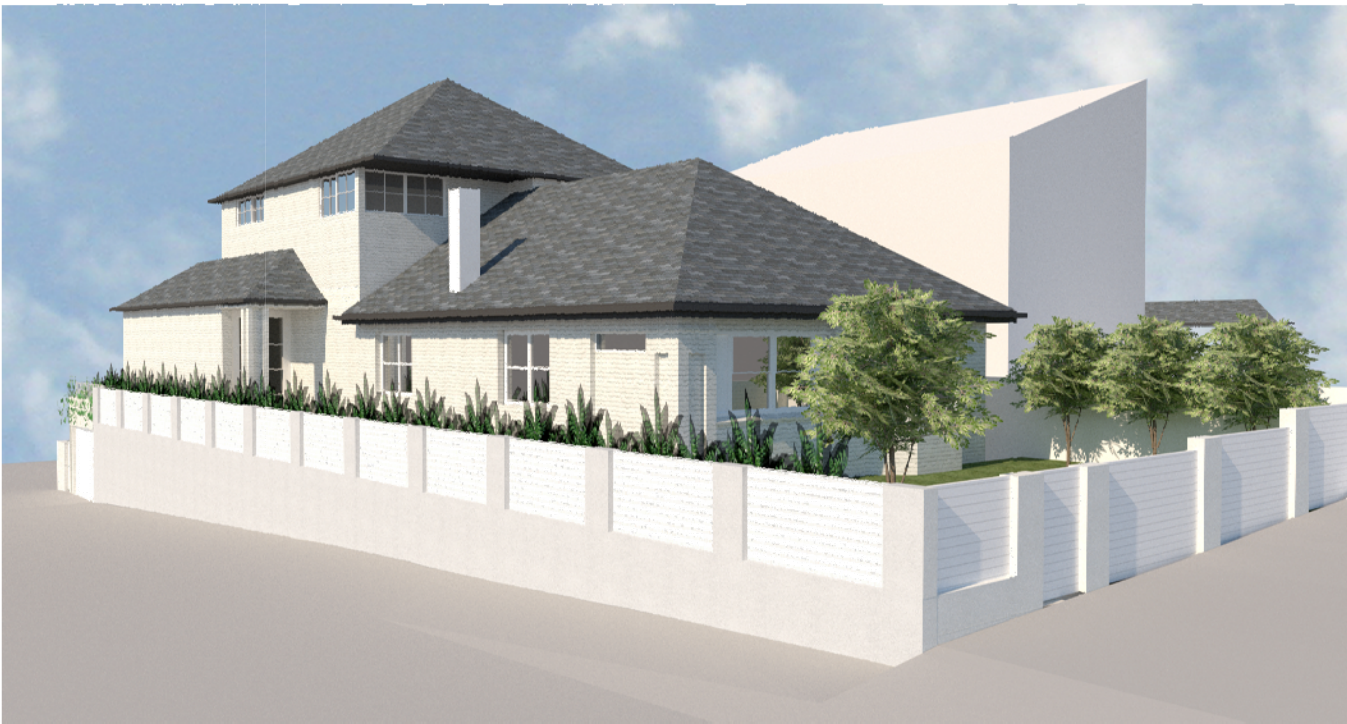
REAR EXTENSION, LOOKING SOUTH-EAST, FROM WHITTLE AVE
