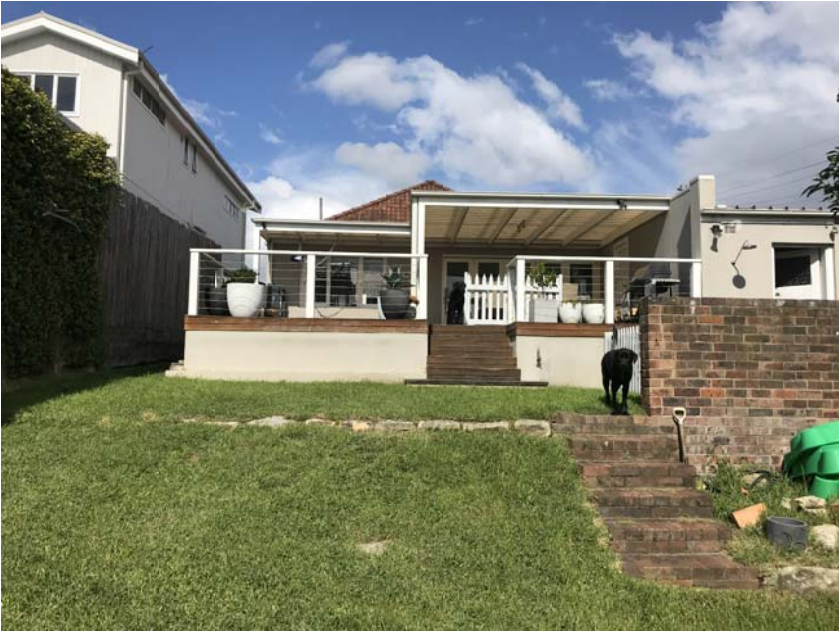
REAR YARD, 28 ETHEL ST, LOOKING SOUTH
