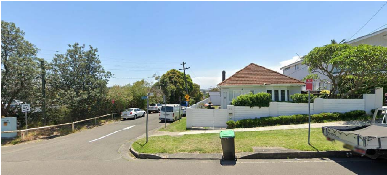
LOOKING NORTH AT 28 ETHEL ST, FROM ETHEL ST
