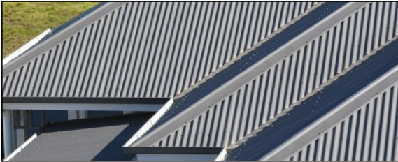
MT-01 PAINTED COLOURBOND METAL ROOF SHEETING. 'IRONSTONE' OR SIMILAR TO MATCH EXISTING. WHERE MARKED ON ELEVATION.
