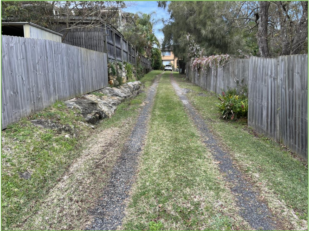
Figure 4: View from where an entering vehicle is required to wait for an egressing vehicle to pass showing the excellent visibility between the two vehicles.
