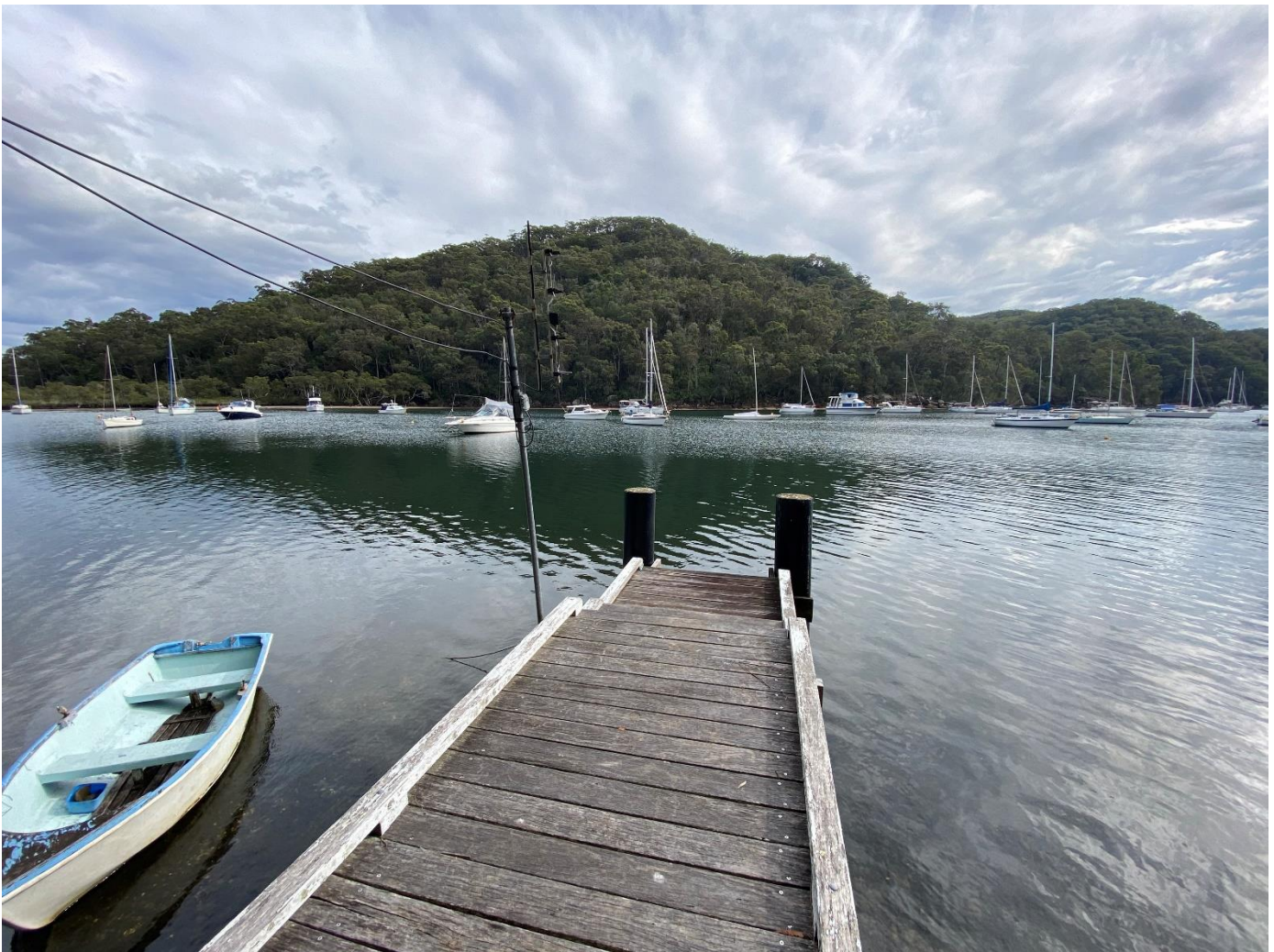
Figure 3: Existing waterfront structures at the Subject Site.
