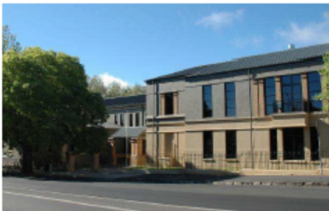
From top: Further new buildings harmonising with the old from different periods and purposes. The height of the first new home is single-storey adjacent to single-storey Victorian neighbours (tip 6). Materials and roof forms reflect surrounding buildings used in subtly different ways to distinguish the new buildings from the old (tip 5); The second is a new building adjoining a historic warehouse and Victorian hotel in Surry Hills; Last two are Orange Courthouse's rear additions continuing the old building's materials and building forms (tips 4 & 6).
