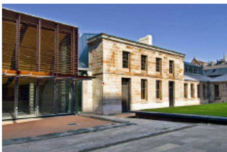
From top: Walsh Bay Wharves, c.1921, once a major shipping port, now a vibrant apartment, theatre and restaurant precinct; Burberry, Sydney, converted from major bank headquarters, c.1925; Burberry interiors re-using bank tellers, seats and desks; The Mint, Sydney, c.1855, where colonial coins were made, now offices.
