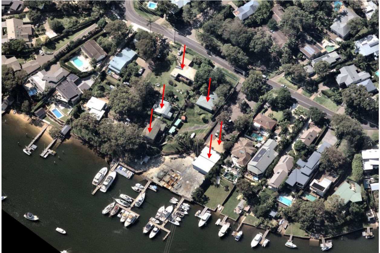
Figure 2: Oblique aerial view of subject properties (main structures at arrows) on 5 April 2022, facing NE
