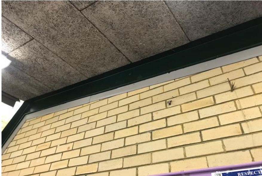
Photograph 9: B00F, R1005 - Art Learning Space, steel beams, undercoat beneath green paint, positive for lead.
