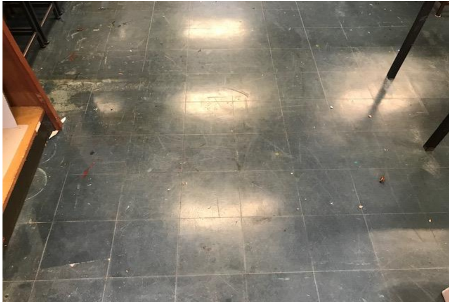
Photograph 7: B00F, R1005 - Art Learning Space, flooring, vinyl tiles, asbestos detected by analysis.
