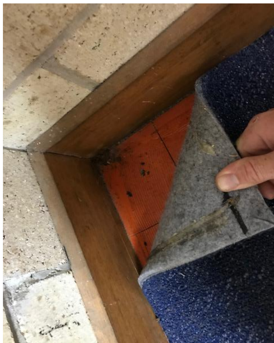
Photograph 13: B00A, R1033 - Classroom, floor, vinyl tiles, asbestos detected by analysis
