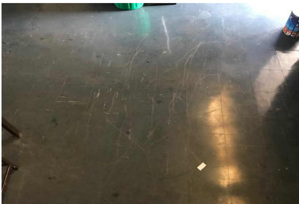
Photograph 4: B00F, R1001 - Art Learning Space , flooring, vinyl tiles, asbestos detected by analysis.
