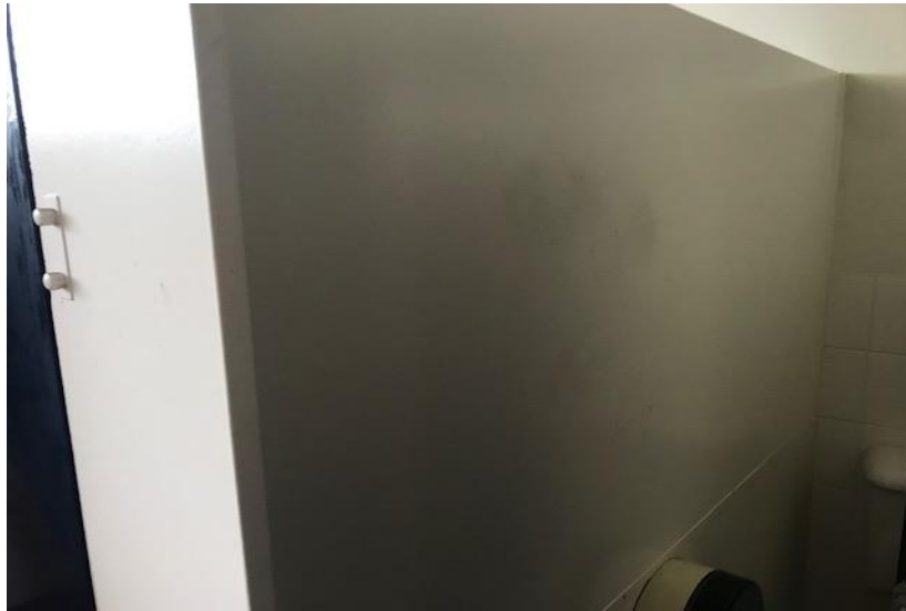
Photograph 5: B00G, R0026 - Girls toilet, cubicle partitions, compressed fibre cement sheet, asbestos detected by analysis
