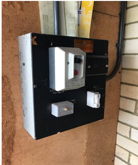
Photograph 11: B00F, R1009 - Plant, electrical backing board, backing board, asbestos detected by analysis.
