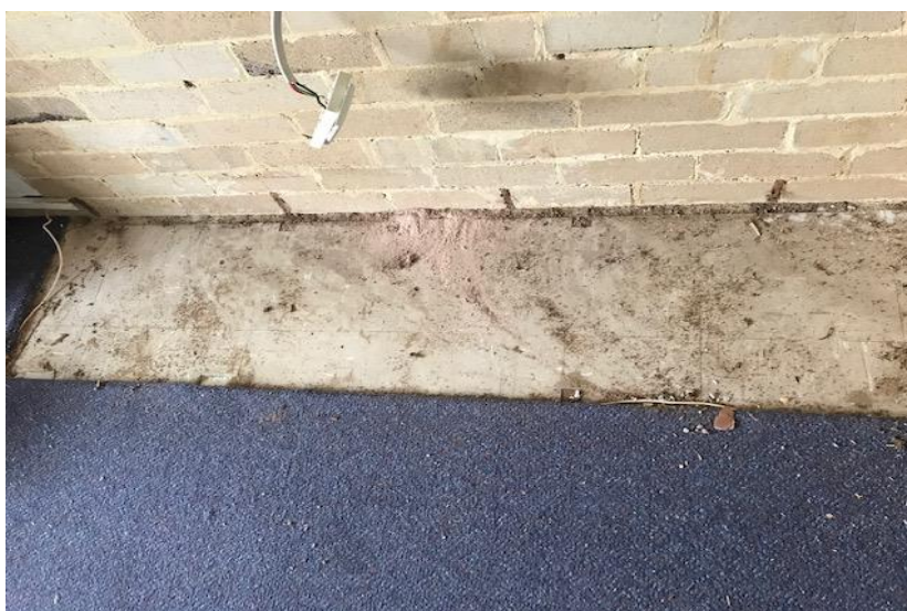
Photograph 5: B00E, R2012 - Office store , floor, vinyl tiles, no asbestos detected by analysis.
