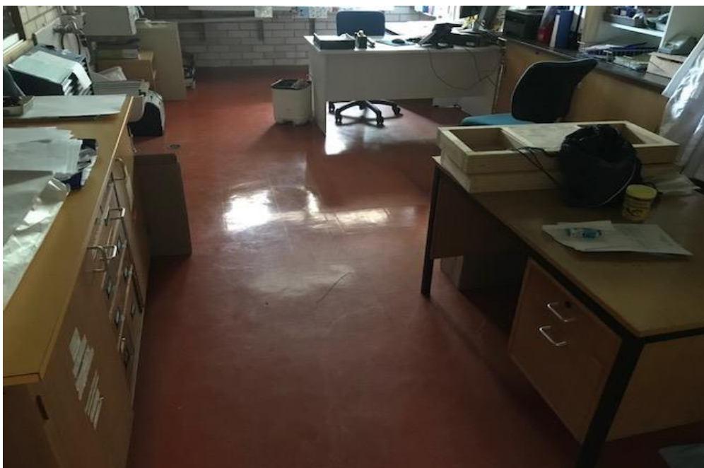
Photograph 11: B00B, R1004 - Office/store, floor, vinyl tiles, asbestos detected by analysis.
