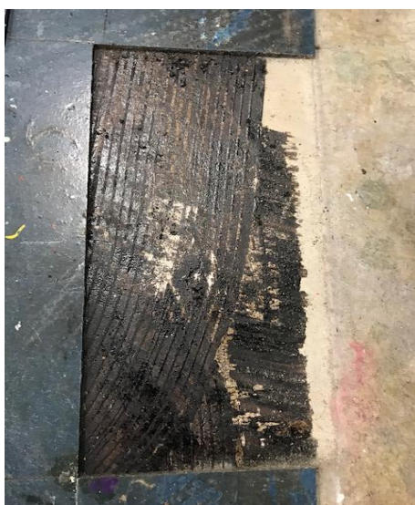
Photograph 5: B00F, R1001 - Art Learning Space , flooring, glue under vinyl tiles, non-asbestos (assumed).
