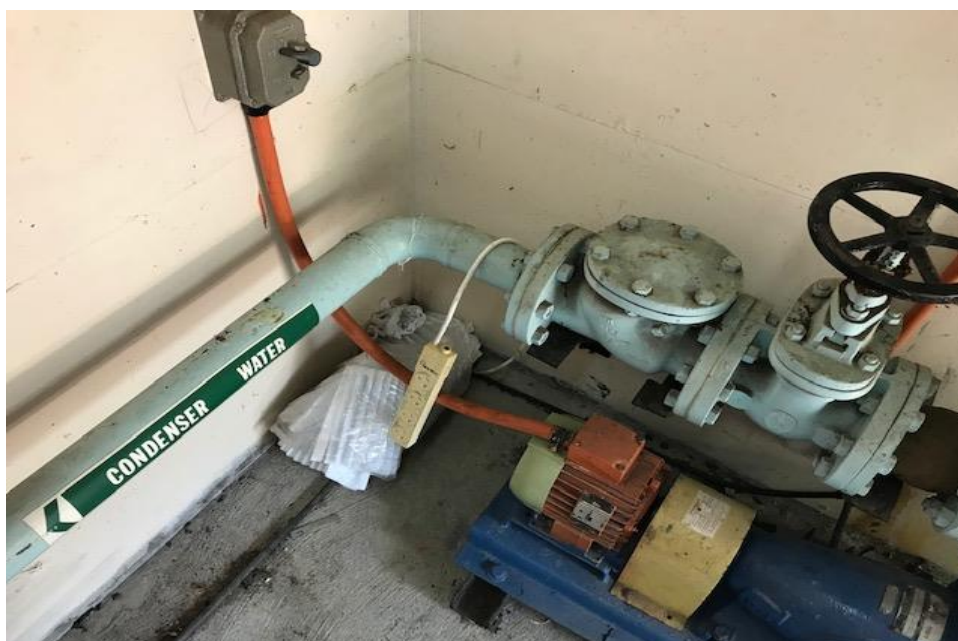
Photograph 8: B00D, R0002 - Plant, pipework, typical blue paint, positive for lead.
