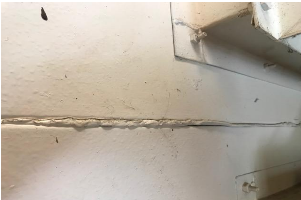
Photograph 1: B00D, throughout, air handling ductwork , mastic to duct, asbestos detected by analysis.
