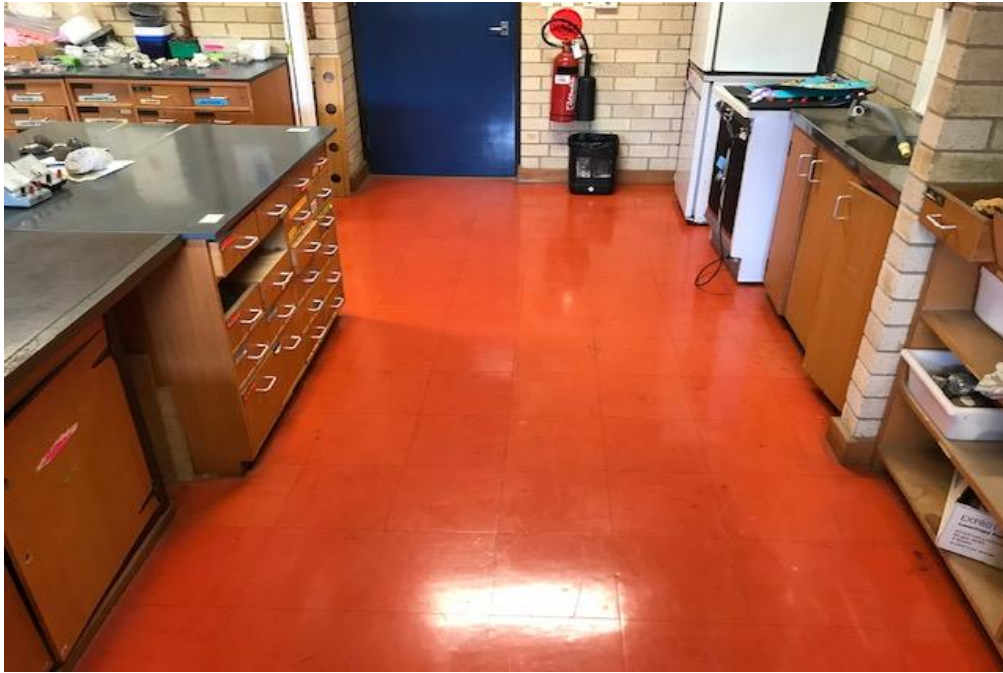
Photograph 19: B00B, R1020 - Preparation Room, floor, vinyl tiles, asbestos (assumed).
