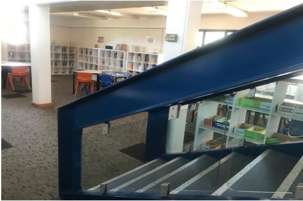
Photograph 3: B00D, R0011 - Main area, handrails, typical blue paint, negative for lead.
