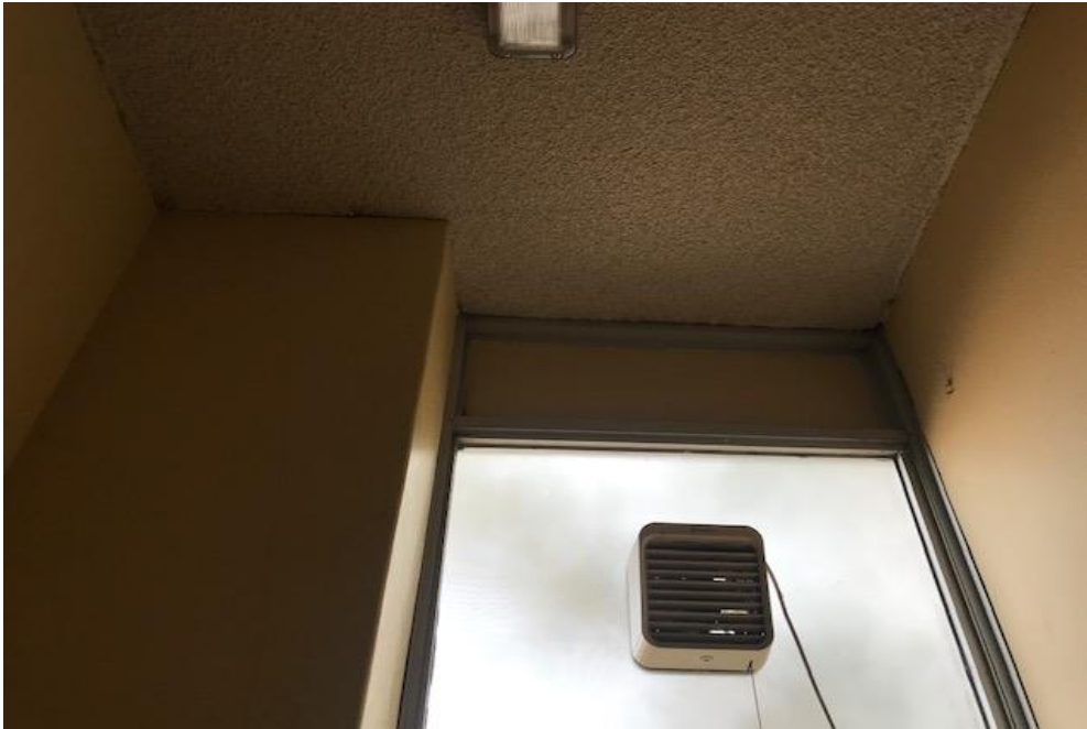
Photograph 3: B00E, R1012 - Staff Female Toilet, ceiling , vermiculite , refer Summary Recommendation.
