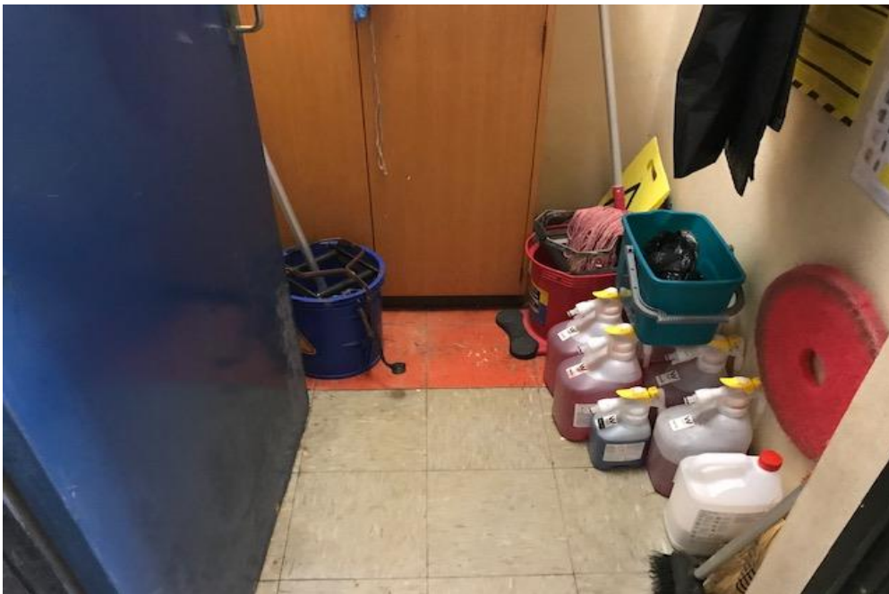
Photograph 2: B00B, R0003 - Cleaning Store, floor, vinyl tiles, asbestos detected by analysis.
