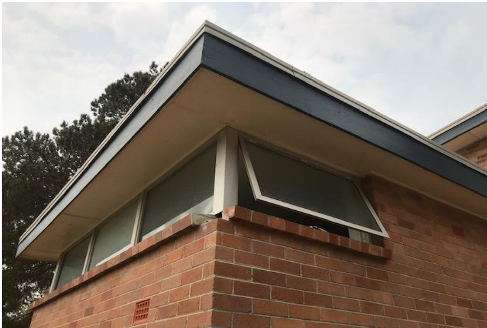
Photograph 4: B00G, exterior, north, south, east and west eave linings, flat fibre cement sheet, asbestos detected by analysis
