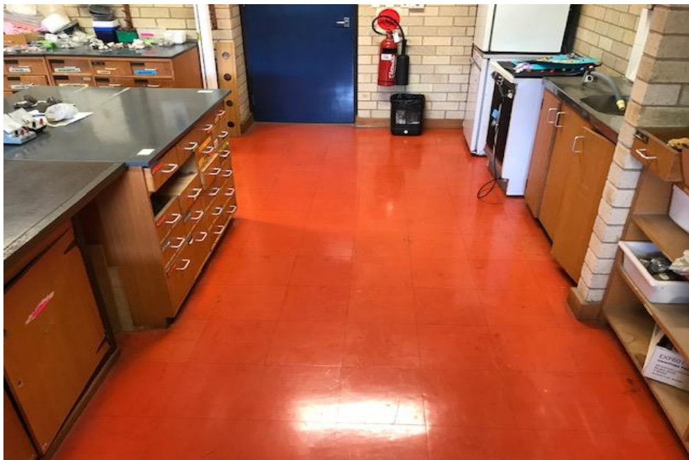
Photograph 14: B00B, R1009 - Preparation Room, floor, vinyl tiles, asbestos detected by analysis.
