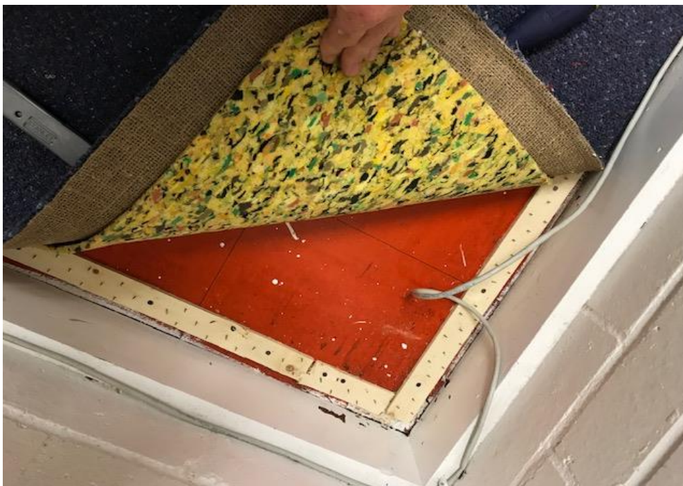
Photograph 3: B00A, R0013 - Design Room, floor, vinyl tiles, asbestos detected by analysis.
