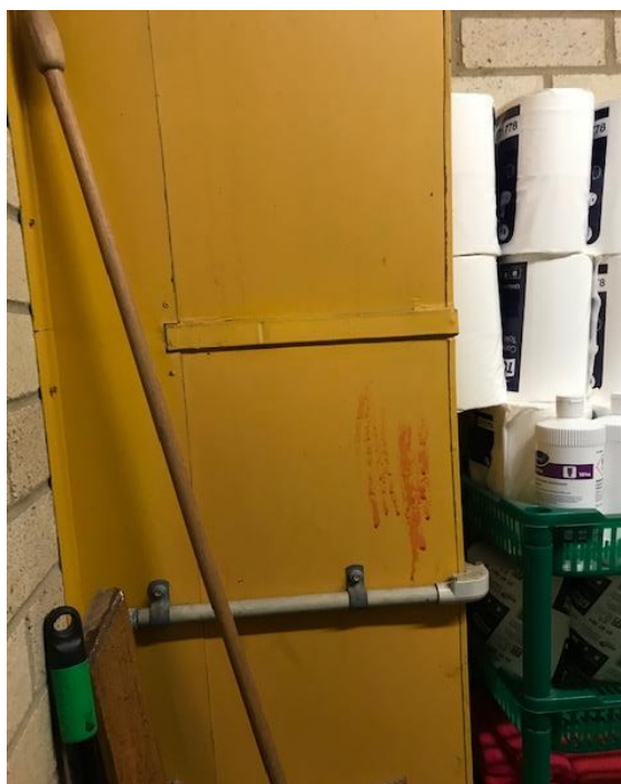
Photograph 12: B00A, R1023 - Plant , air handling duct work, yellow paint, positive for lead.
