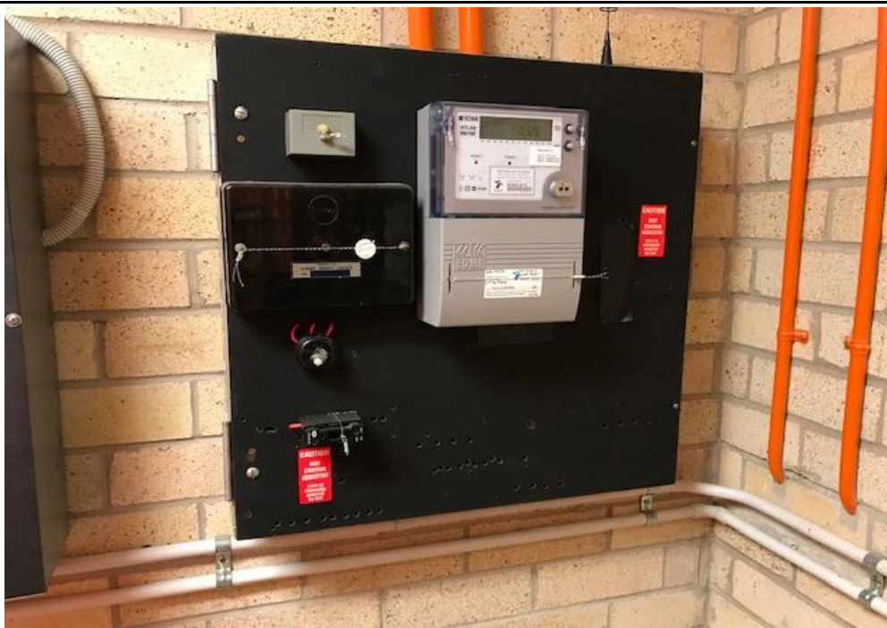
Photograph 5: B00A, R0019 - Main switchboard, electrical backing board, flat fibre cement sheet, asbestos (assumed).
