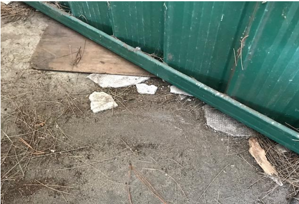
Photograph 2: B00G, exterior, south eastern corner of building, on floor, fibre cement debris, no asbestos detected by analysis
