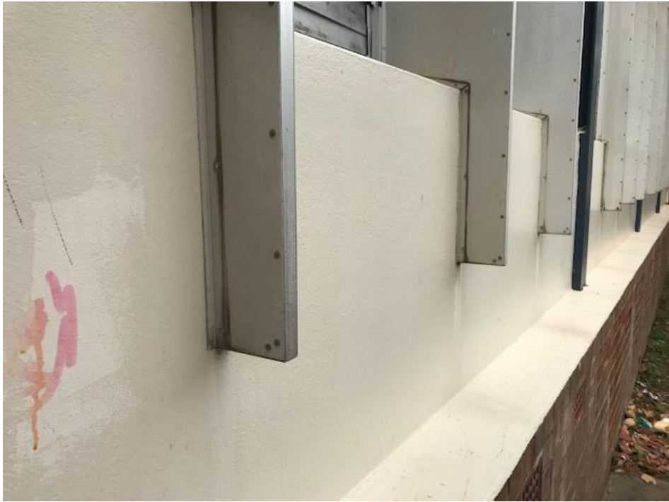
Photograph 1: B00G, exterior, walls, cream paint, positive for lead
