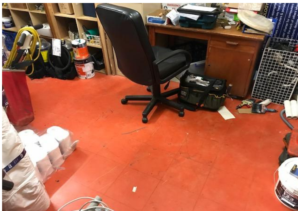
Photograph 6: B00A, R0022 - Sports Equipment Store , floor, vinyl tiles, asbestos detected by analysis.
