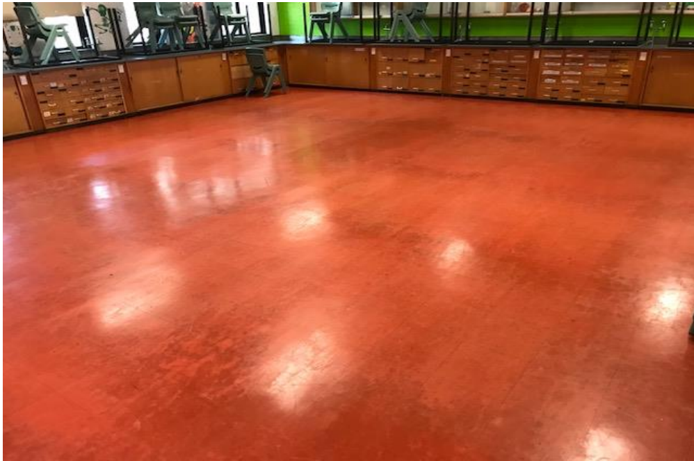
Photograph 17: B00B, R1012 - Laboratory, floor, vinyl tiles, asbestos (assumed).
