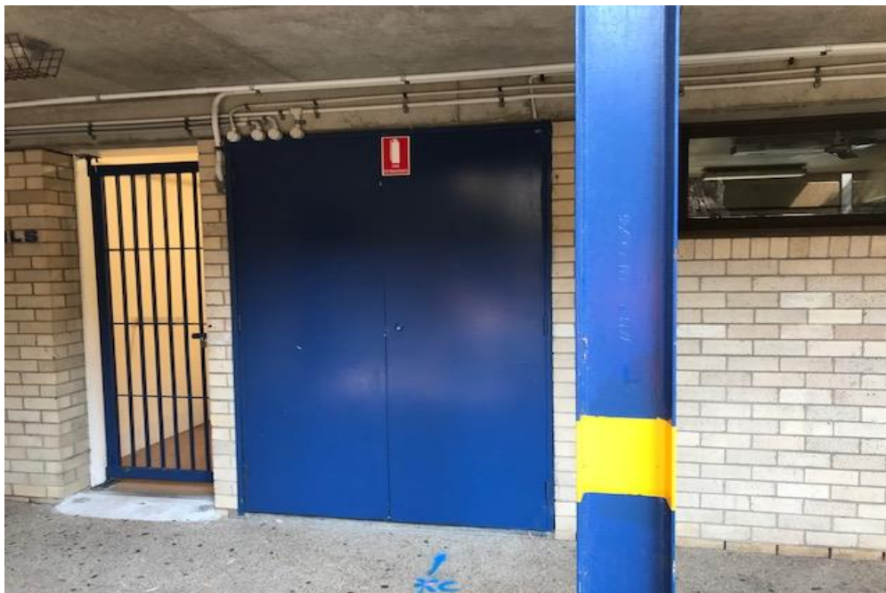
Photograph 6: B00C, exterior, throughout, typical blue paint, negative for lead.
