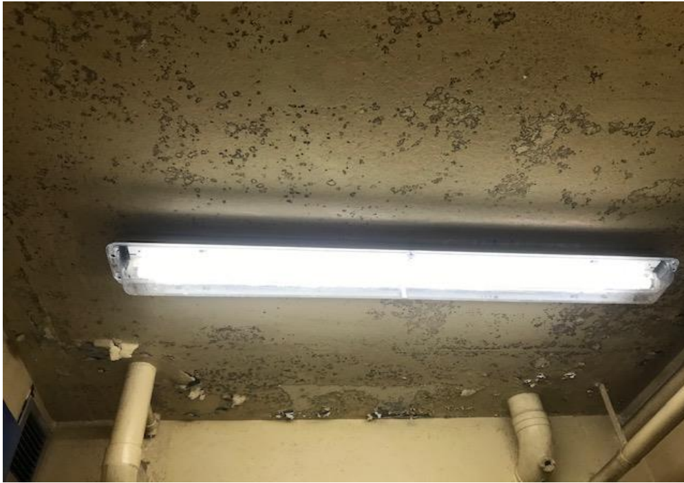
Photograph 1: B00B, R0002 - Staff Toilet, ceiling, yellow paint, positive for lead.
