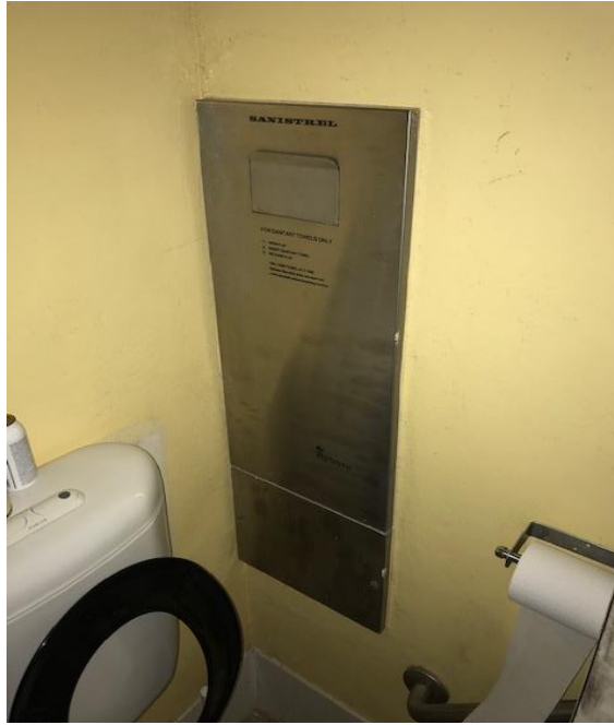
Photograph 9: B00B, R1002 - Staff Female Toilet, wall, incinerator, internal component(s), asbestos (assumed).
