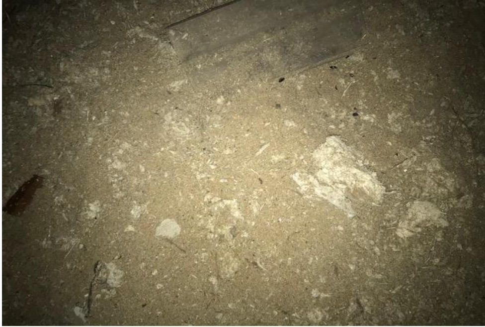
Photograph 3: B00G, exterior, subfloor, throughout, loose fibre in sand/soil, asbestos detected by analysis
