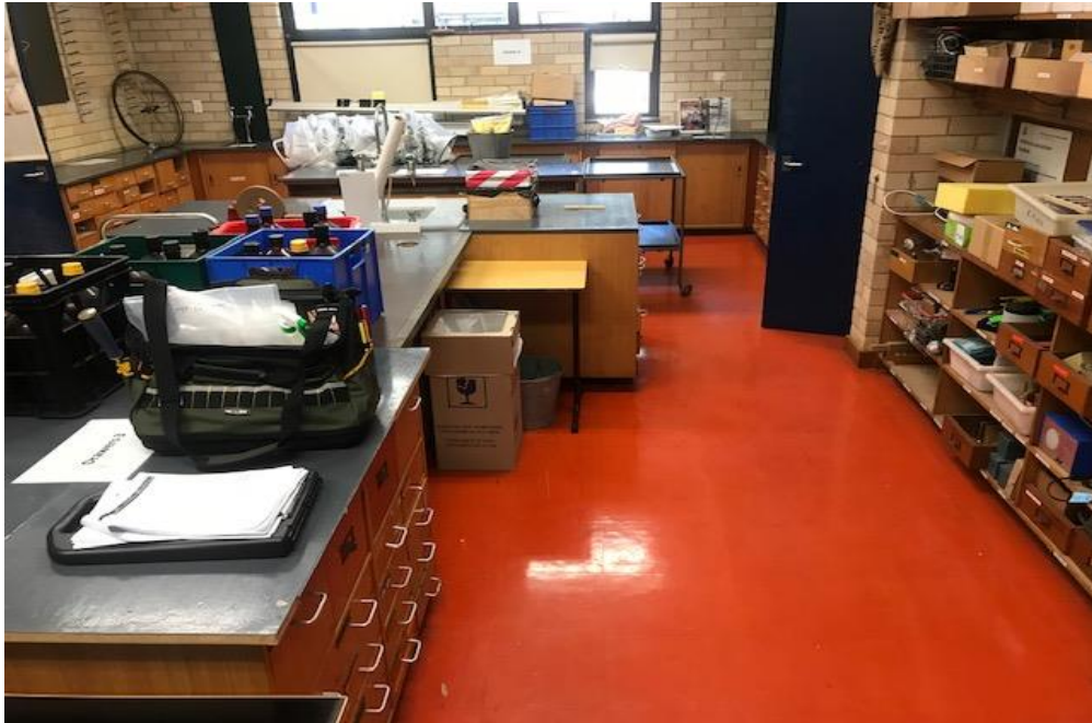
Photograph 5: B00B, R0012 - Preparation Room, floor, vinyl tiles, asbestos detected by analysis.
