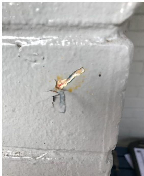
Photograph 12: B00F, exterior, brickwork, throughout, undercoat to grey paint, positive for lead.
