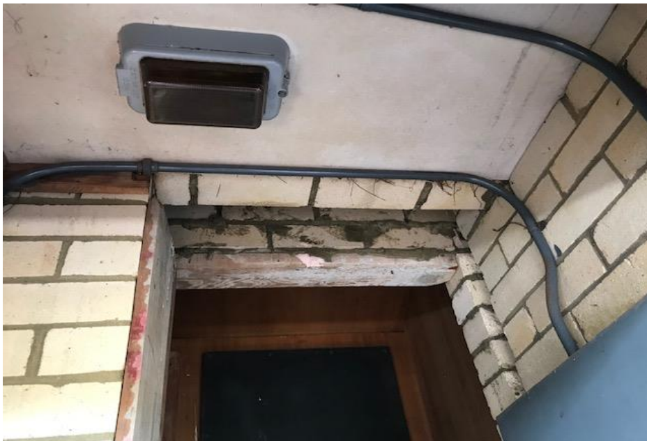
Photograph 10: B00F, R1009 - Plant , ceiling structure / lining , fibre cement sheet, asbestos detected by analysis.
