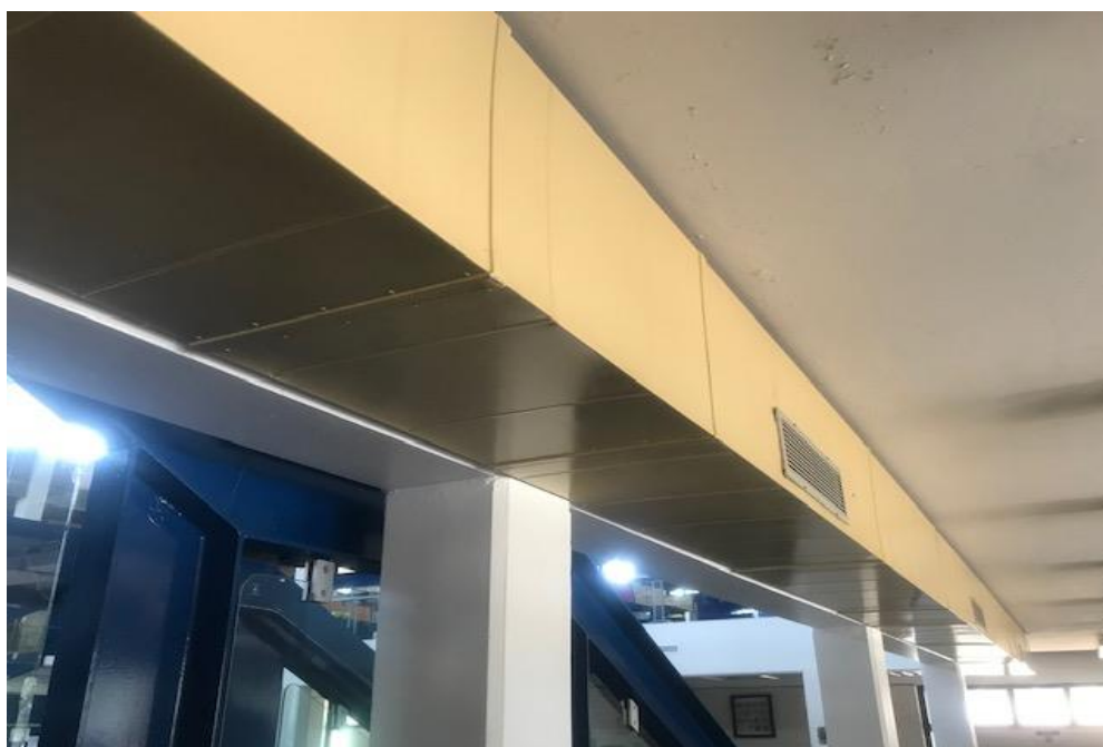
Photograph 2: B00D, R0011 - Main area, air handling ductwork , cream paint , positive for lead.
