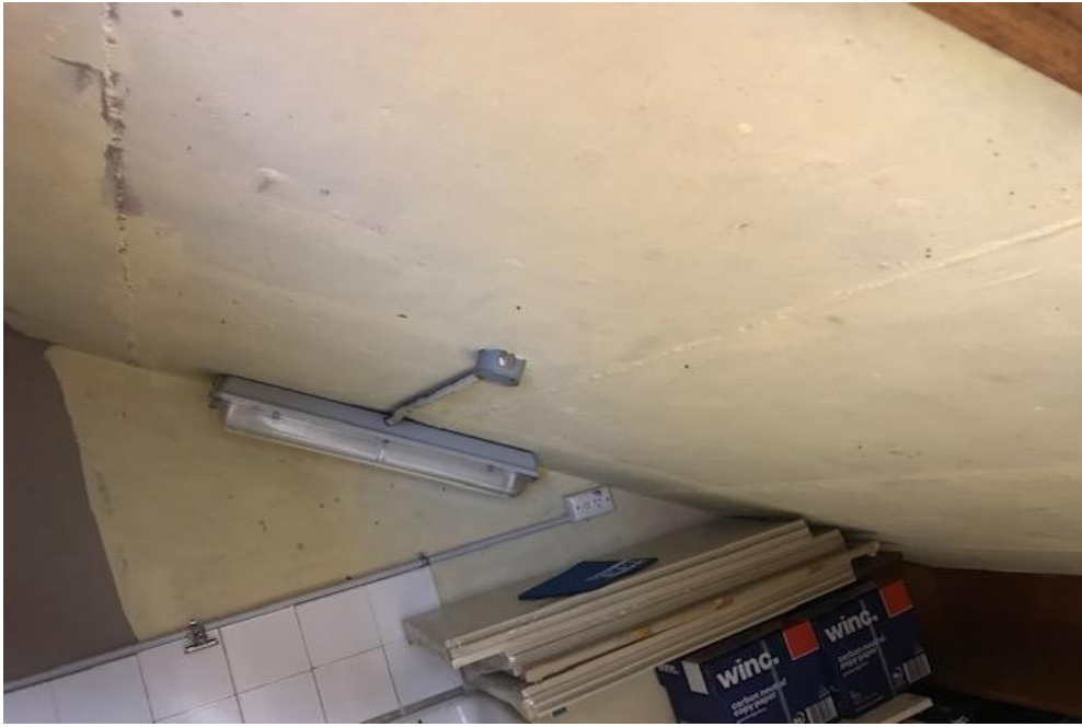
Photograph 1: B00E, R0014 - Storeroom, ceiling , vermiculite, appears removed.
