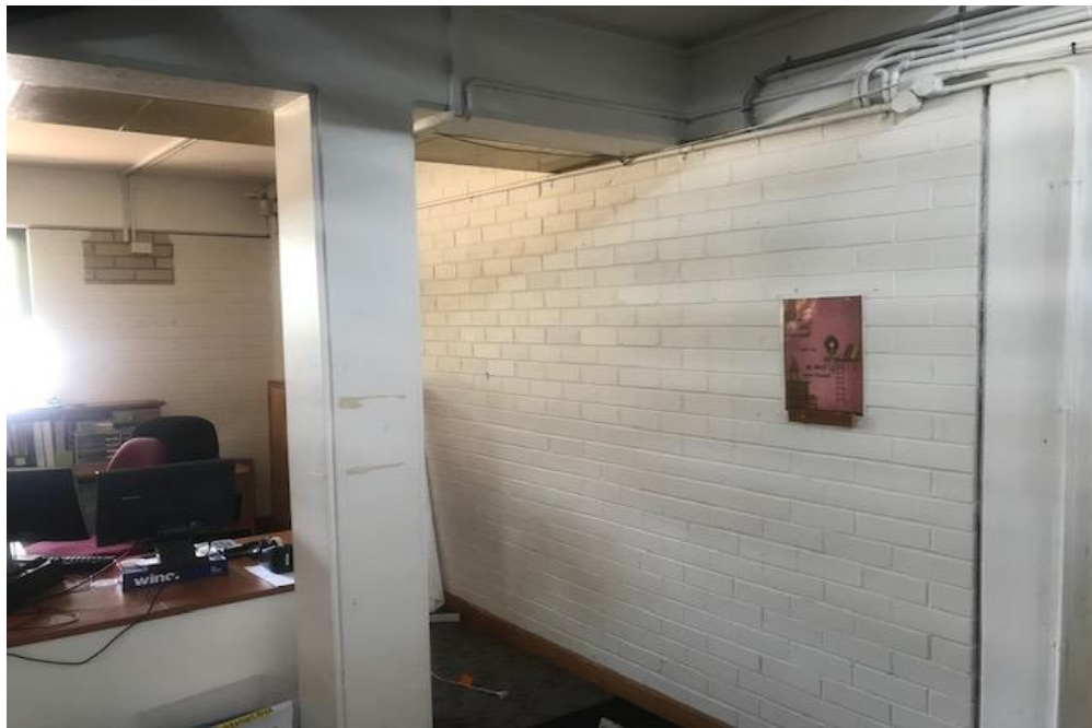
Photograph 4: B00D, internal, throughout, walls, typical white paint, negative for lead.
