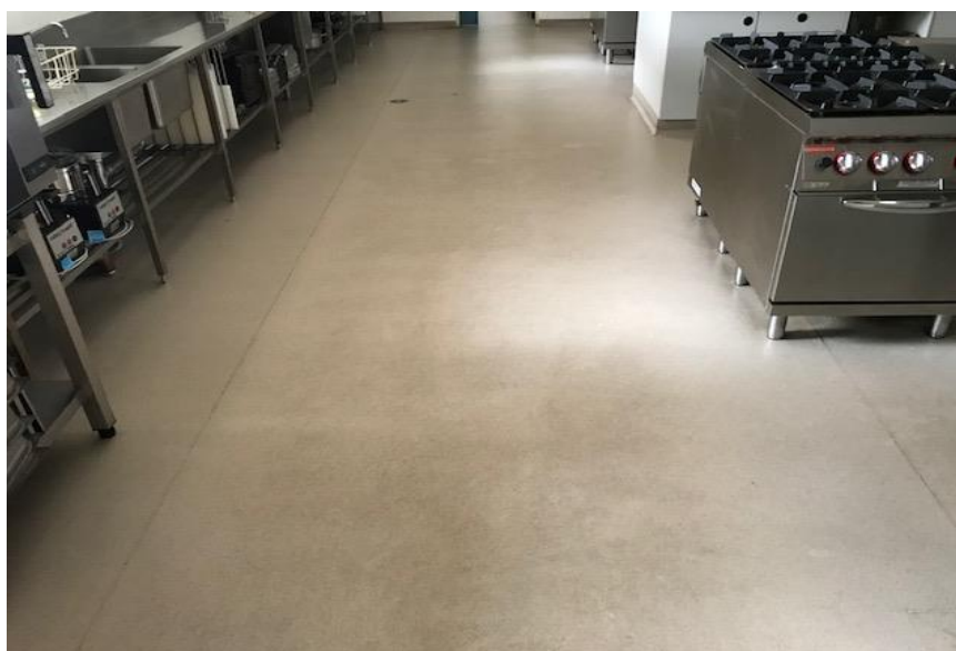
Photograph 16: B00A, R1001 - Food Technology, floor, vinyl tiles, asbestos detected by analysis
