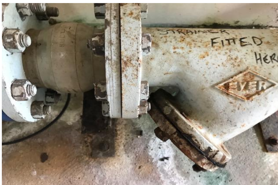
Photograph 7: B00D, R0002 - Plant, pipework, gasket, no asbestos detected by analysis.
