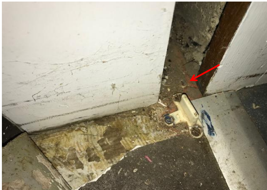
Photograph 2: B00A, R0010 - Design Room , floor (below newer floor covering/s), residual vinyl tile and/or associated debris, asbestos detected by analysis
