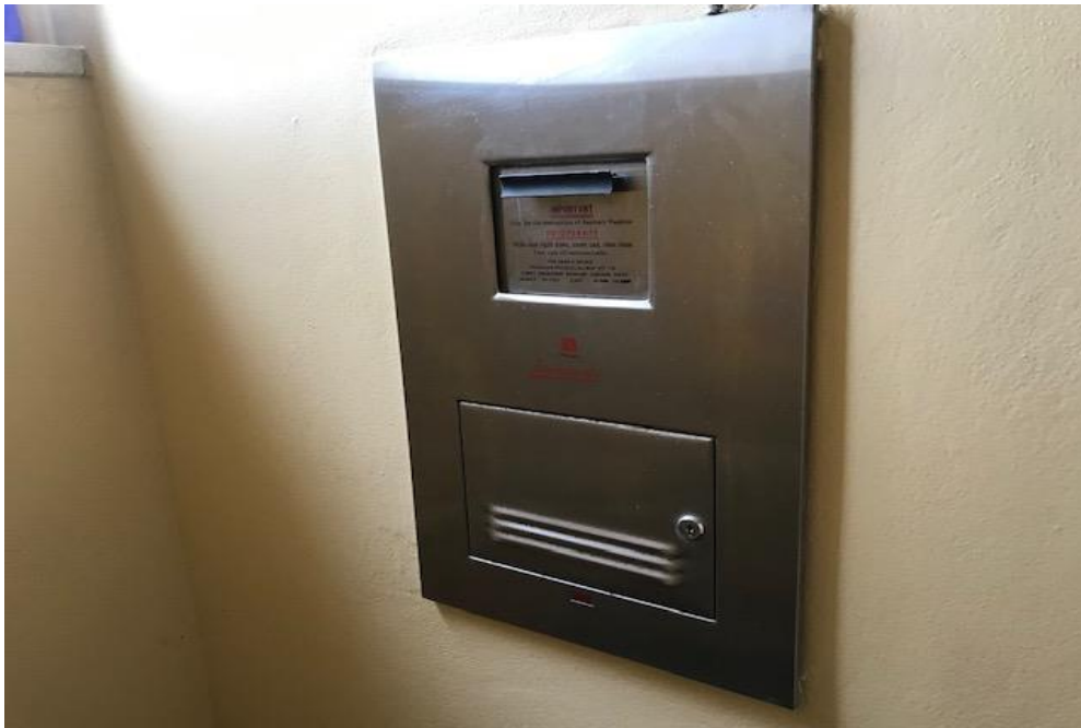
Photograph 2: B00E, R1012 - Staff Female Toilet, incinerator on wall, internal insulation and/or other components, asbestos (assumed).
