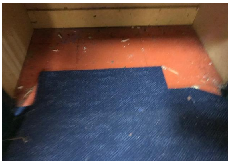
Photograph 15: B00A, R1034 - Control Room, floor, vinyl tiles, asbestos detected by analysis
