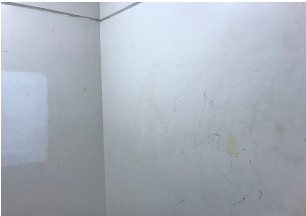
Photograph 7: B00A, R0052 - Shower and Toilets, walls, typical grey paint, negative for lead.
