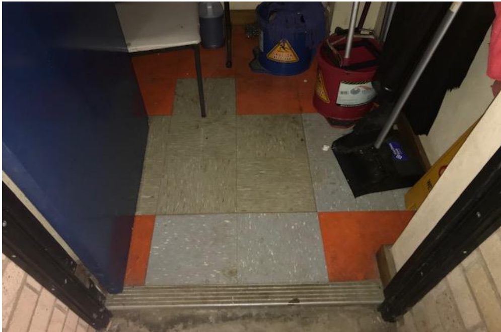
Photograph 10: B00B, R1003 - Cleaning Store , floor, vinyl tiles, asbestos detected by analysis.
