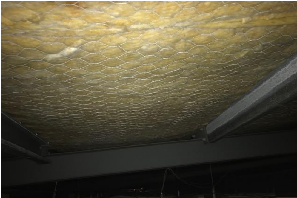
Photograph 7: B00C, first floor, ceiling cavity, insulation , SMF identified visually.
