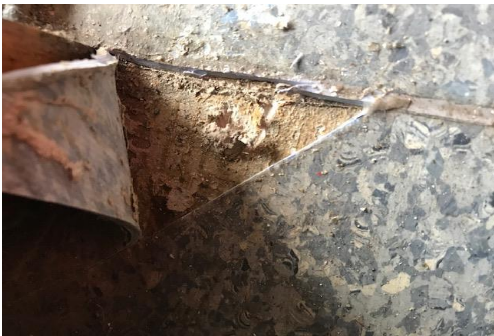
Photograph 2: B00F, R0010 - Art Learning Space , flooring, vinyl and underlay , non asbestos (assumed).
