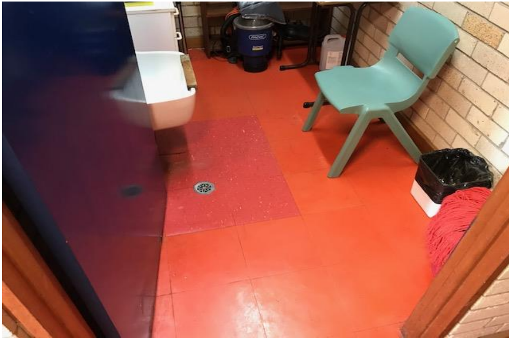
Photograph 5: B00C, R1017 -Cleaning Store , floor, vinyl tiles, asbestos detected by analysis.
