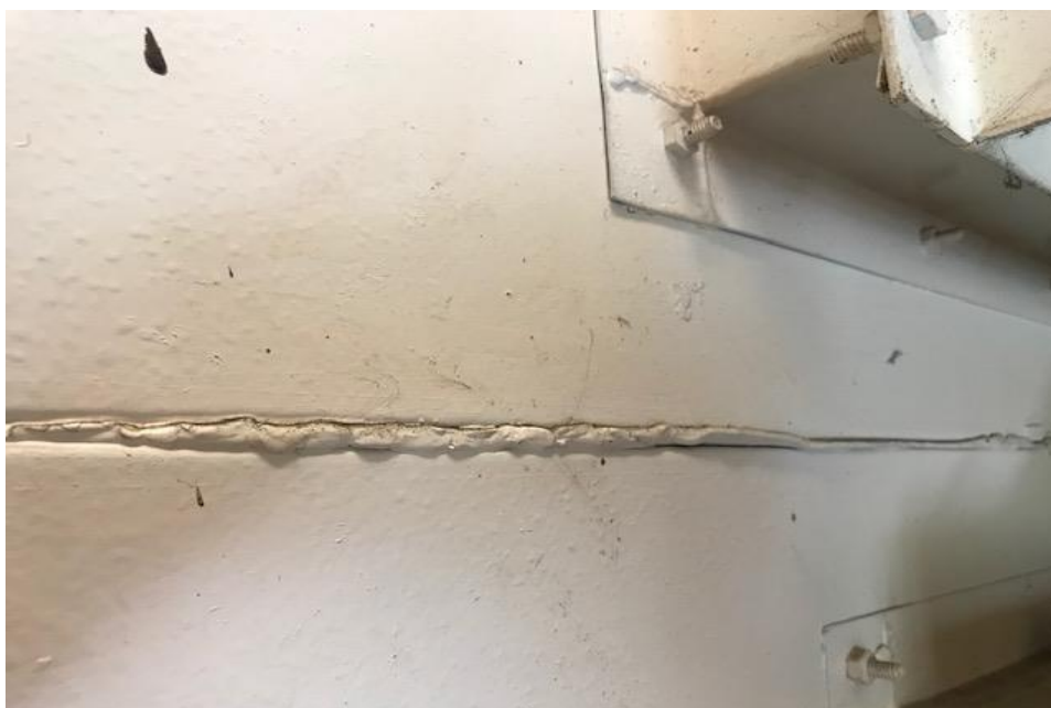
Photograph 8: B00E, R2019 - Plant Room, air handling duct work, mastic to duct, asbestos detected by analysis.
