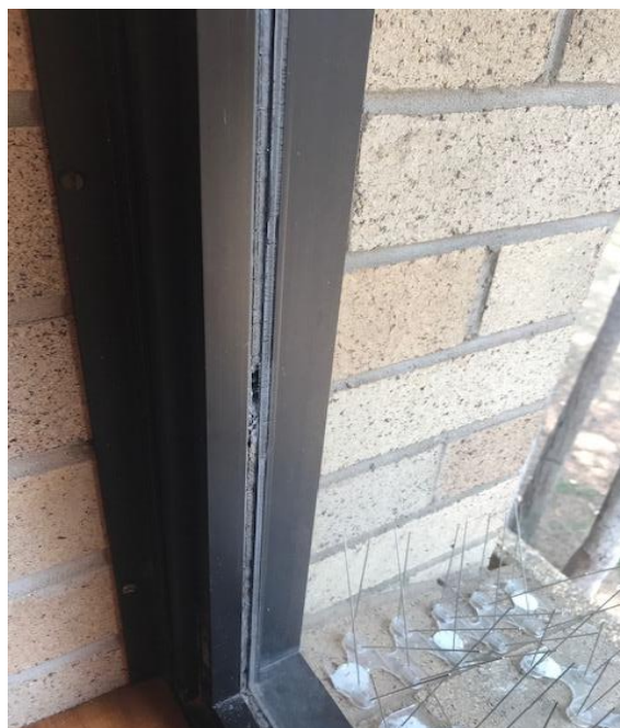
Photograph 5: B00D, internal, throughout, windows, mastic, asbestos detected by analysis.
