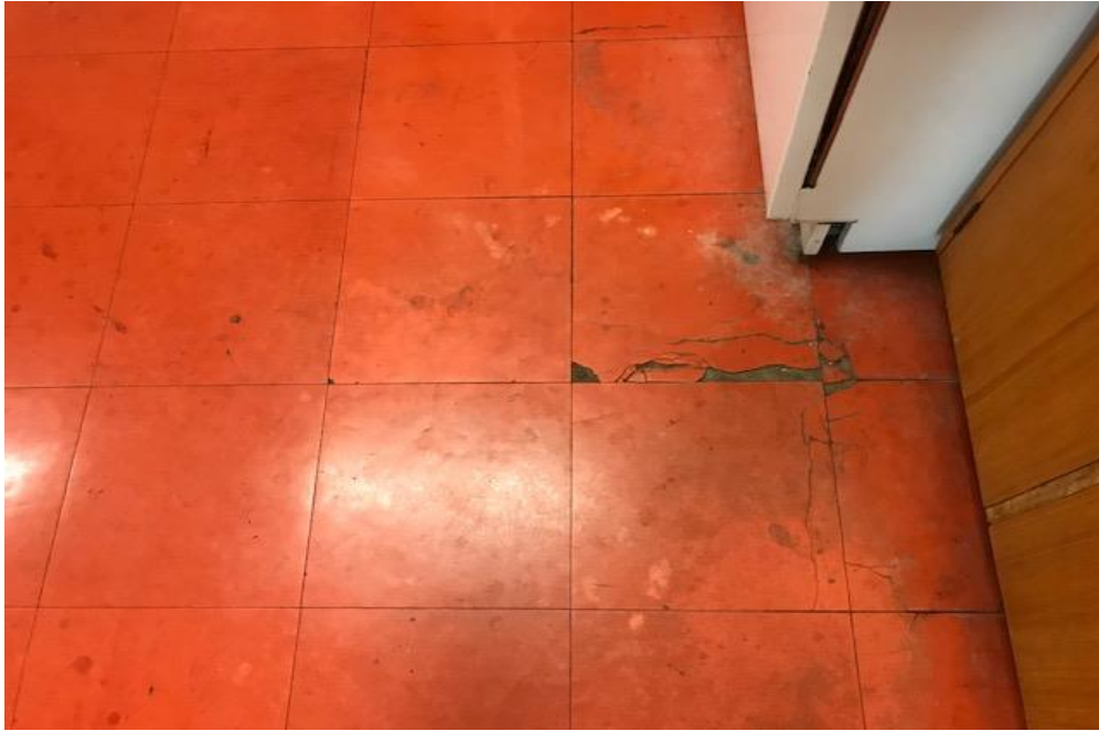
Photograph 13: B00B, R1007 - Laboratory, floor, vinyl tiles, asbestos detected by analysis.
