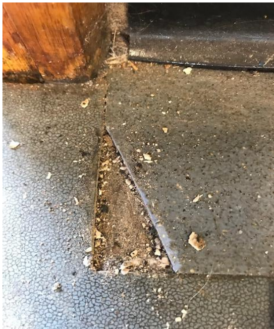
Photograph 1: B00F, R0003 - Art Learning Space, flooring, vinyl and underlay , no asbestos detected by analysis.
