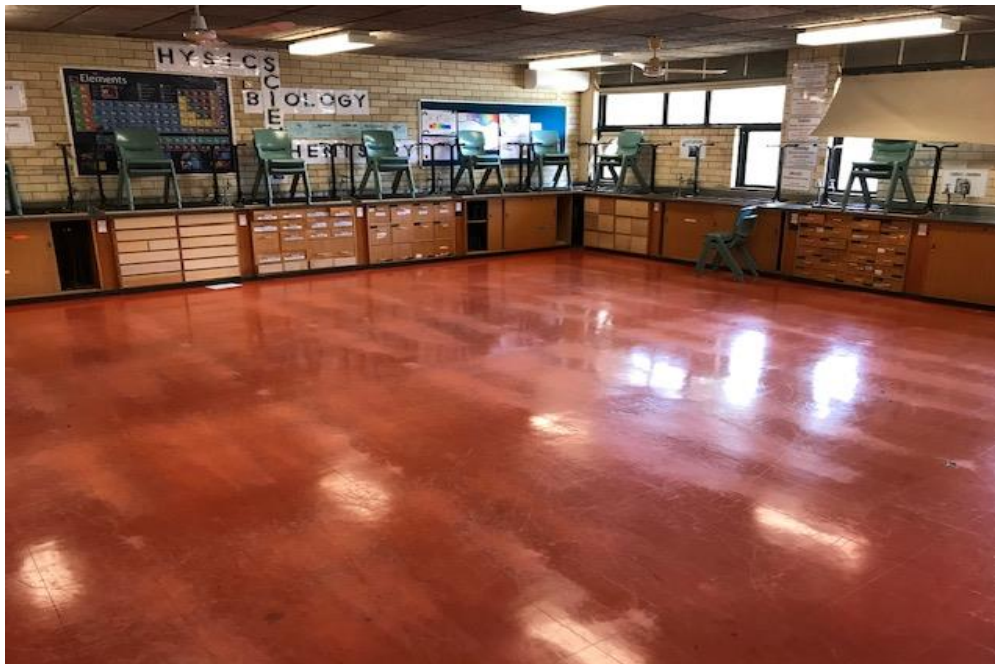
Photogrtaph 16: B00B, R1011 - Laboratory, floor, vinyl tiles, asbestos detected by analysis.
