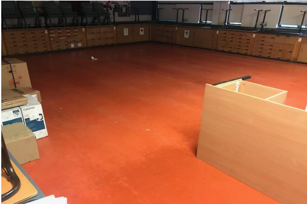
Photograph 7: B00B, R0014 - Laboratory , floor, vinyl tiles, asbestos detected by analysis.
