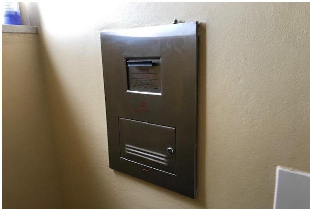
Photograph 4: B00E, R2010 - Staff female toilet , incinerator on wall, internal insulation and/or other components, asbestos (assumed).
