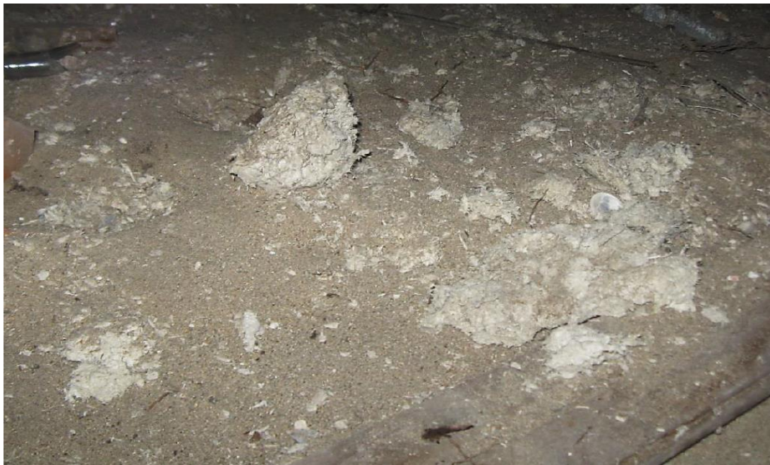
Photograph 6: B00G, exterior, subfloor, throughout, loose fibre in sand/soil, asbestos detected by analysis
