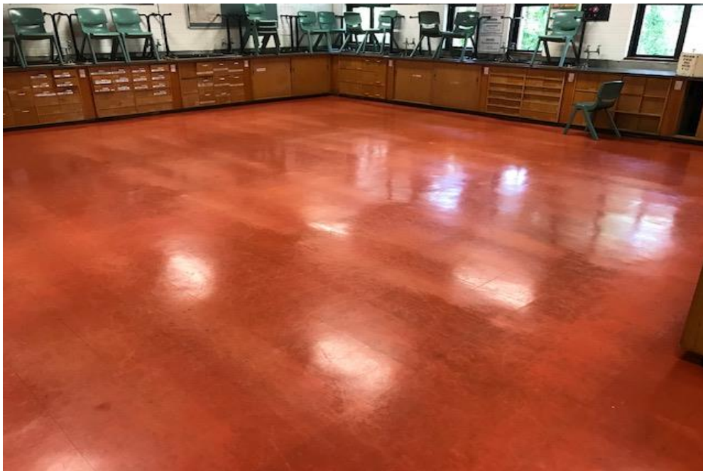
Photograph 18: B00B, R1014 - Laboratory, floor, vinyl tiles, asbestos detected by analysis.
