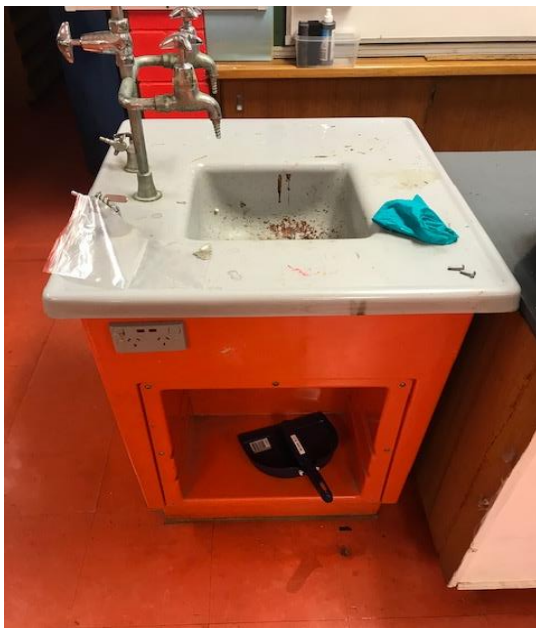
Photograph 8: B00B, R0014 - Laboratory , void under teacher's sink, fibrous debris , asbestos detected by analysis.
