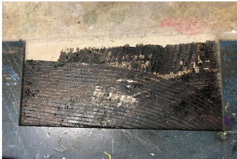
Photograph 8: B00F, R1005 - Art Learning Space , flooring, glue under vinyl tiles, no asbestos detected by analysis.
