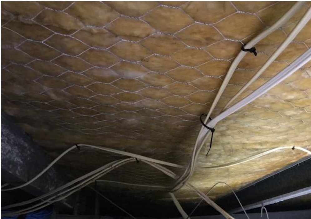
Photograph 9: B00A, Level 1, internal, ceiling voids, insulation, SMF identified visually.
