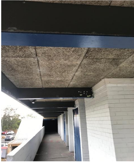
Photograph 13: B00F, exterior, throughout, blue paint, negative for lead.
