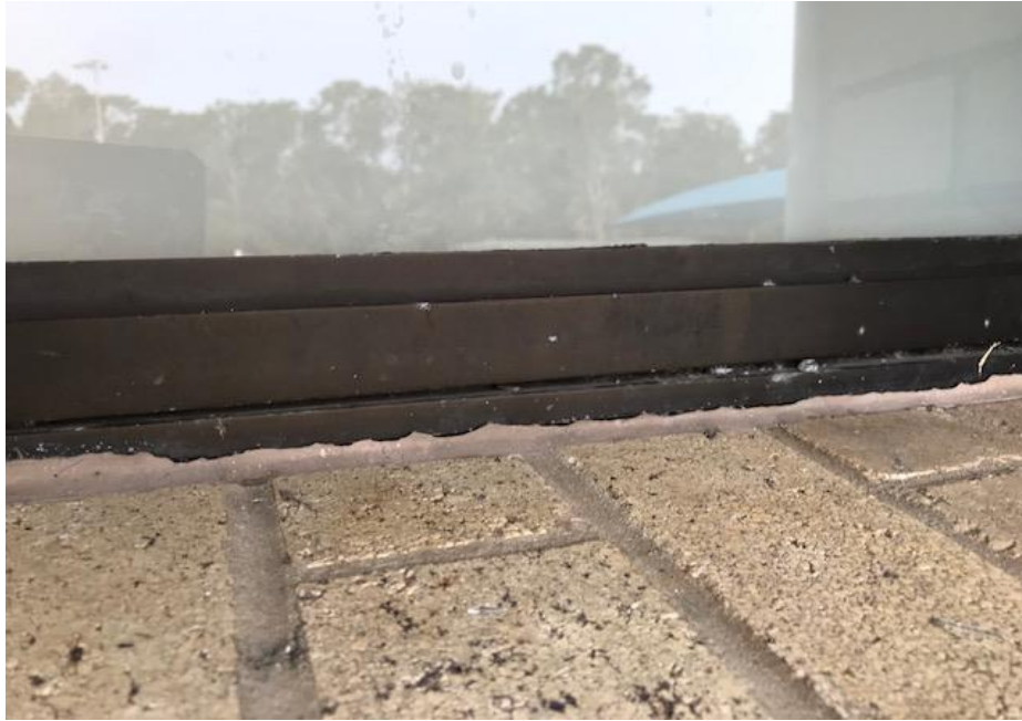
Photograph 1: B00A, throughout , windows, brown putty/mastic , asbestos detected by analysis.
