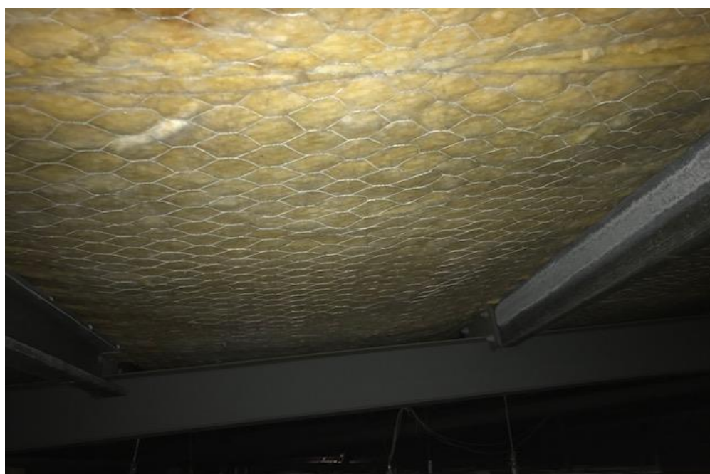
Photograph 6: B00D, internal, level 1 , ceiling cavity, insulation, SMF identified visually.
