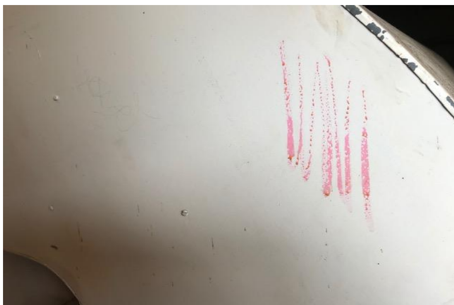
Photograph 7: B00E, R2019 - Plant Room, air handling duct work, white paint, positive for lead.
