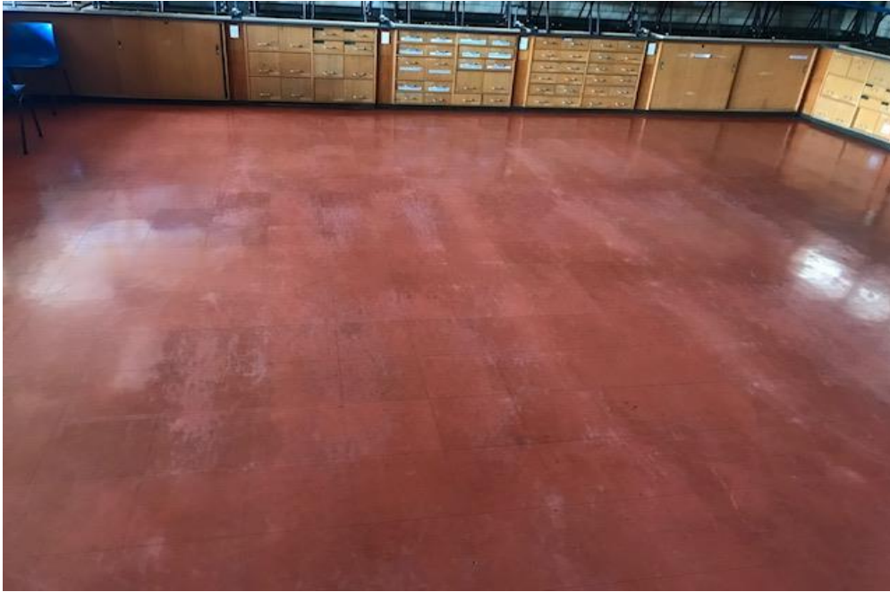
Photograph 15: B00B, R1010 - Laboratory , floor, vinyl tiles, asbestos detected by analysis.
