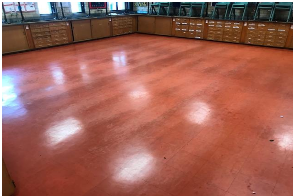
Photograph 4: B00B, R0011 - Laboratory , floor, vinyl tiles, asbestos detected by analysis.
