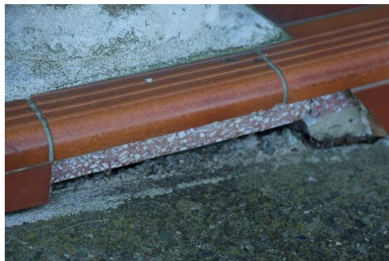
Figure 20. Detail showing the (potentially original) terrazzo tile beneath the modern stairs at the Raglan Street entrance.
