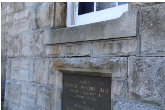
Figure 21 Example of exterior sandstone showing deteriorating mortar.
