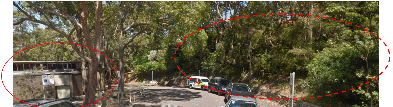
Figure 9: Civic Parade view indicating subject site on right and I 50 (Dee Why Public Library) and I 137 (Civic Centre Landscaping) on left.
