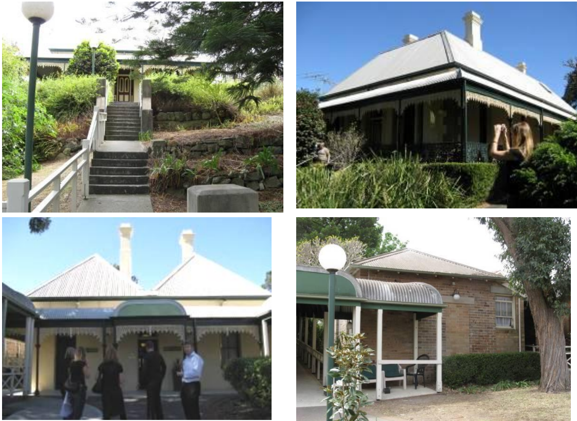
Figure 5: 1892 Pacific Lodge Administration & adjacent c1911 Store / Amenities building
